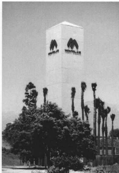
Concealed in an architectural tower
