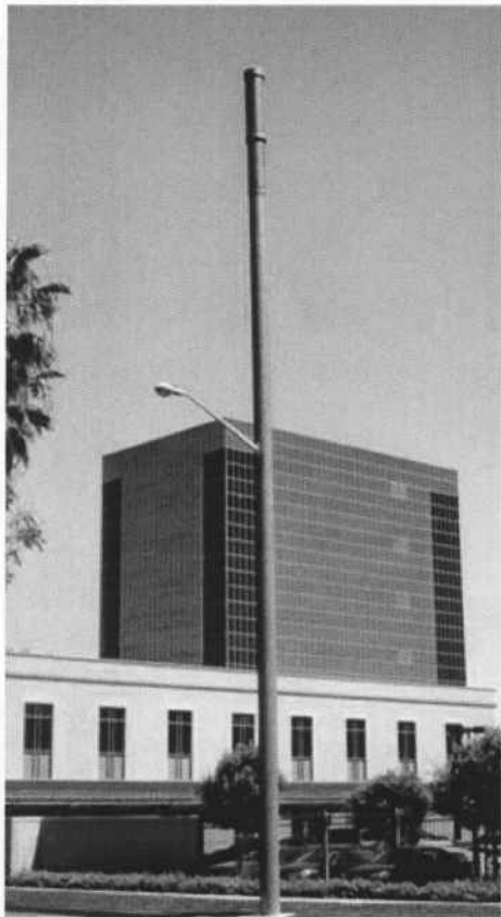
Disguised as a Streetlight
