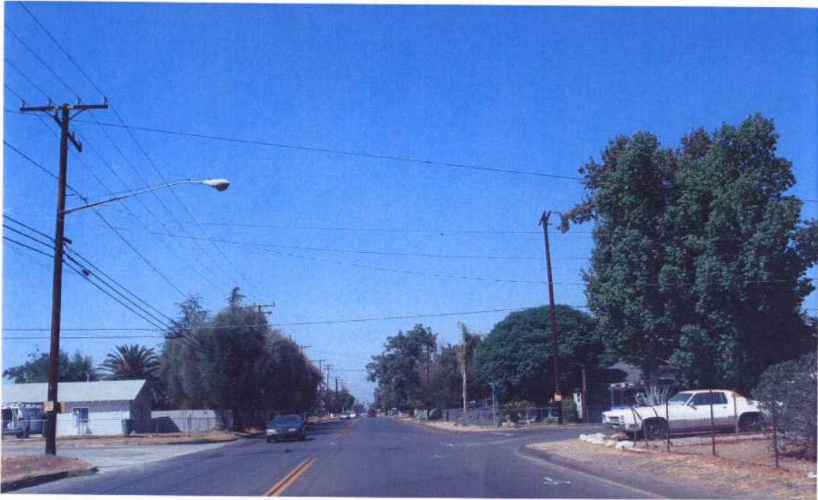
Typical Overhead Utilities on Eastbound Stetson Avenue
