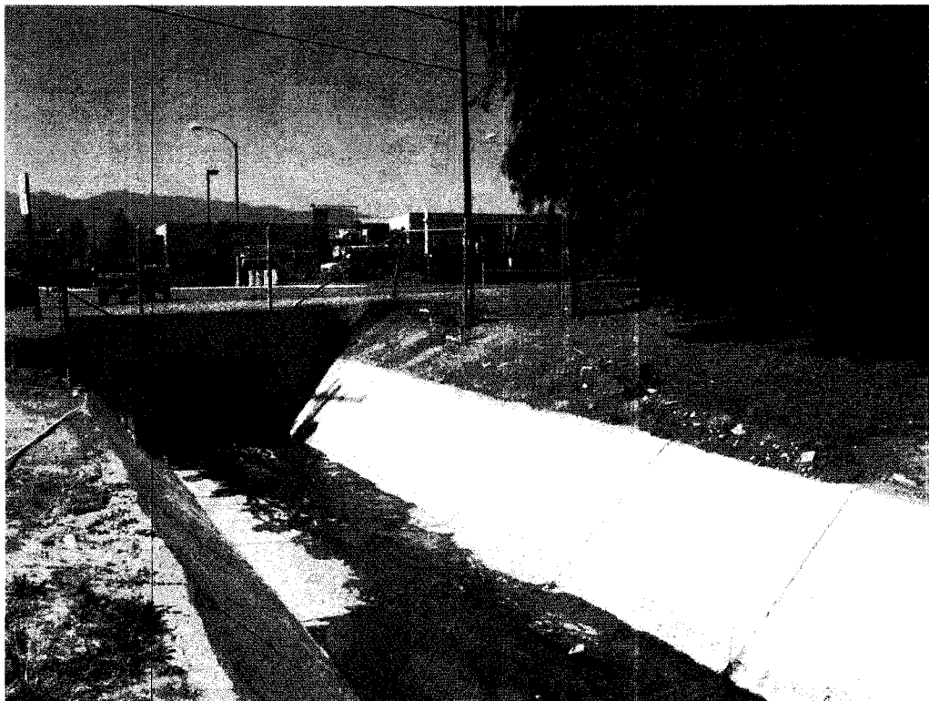
El Cerrito Channel looking west at location of proposed storm drain connection
