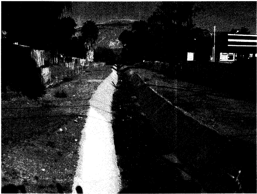
El Cerrito Channel looking northeast at location of proposed storm drain connection
