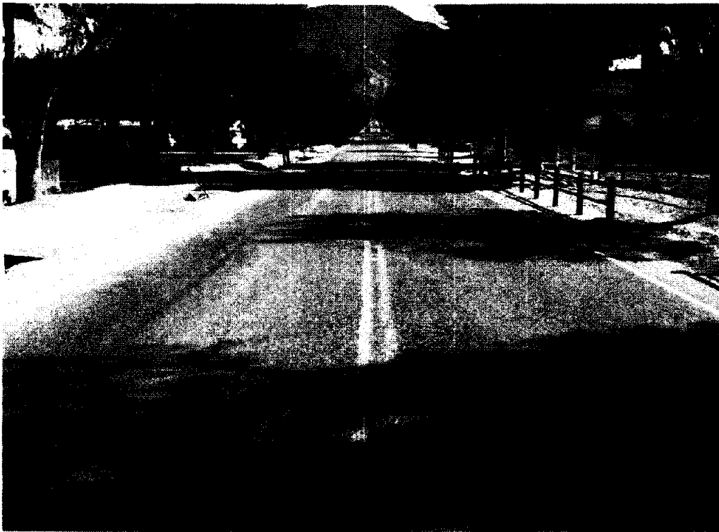
Line N-1, Stage 2: 7 th Street looking east (just west of Pedley Avenue)
