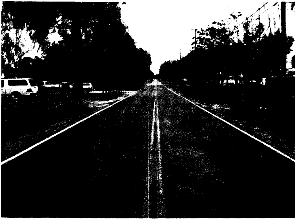
Line NA-3: Pedley Avenue looking north (just north of 5 th Street)
