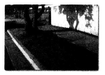
Glen Avon Elementary School and Glen Avon Elementary School South are located within this segment. The roadway; for the most part is improved to full width; however, there is no concrete curb and gutter on the west side of the street. Curb and gutter on the east side of the street is in various levels of disrepair and in some places buckled and raised. The existing curb ramps at Stonewood Lane do not meet current ADA requirements and will be replaced.
