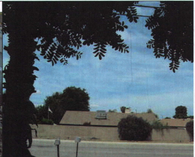
Powerline dropping to the ground in front of dwell KR
