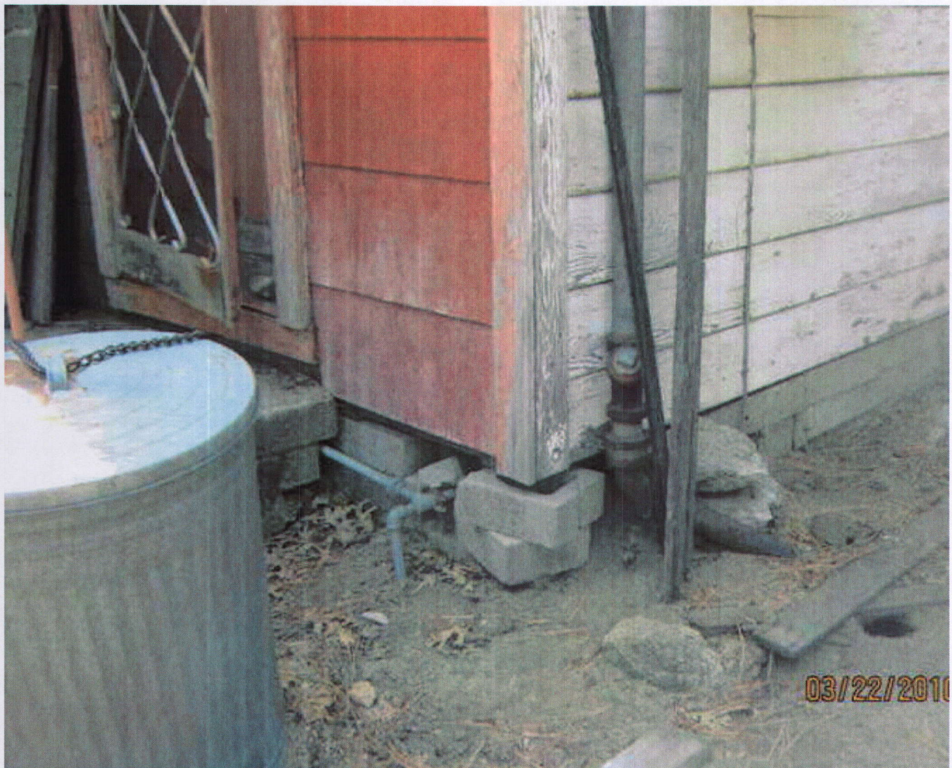
CForrey / Defect #8 Foundation made of unsupported block - 03/22/2010
