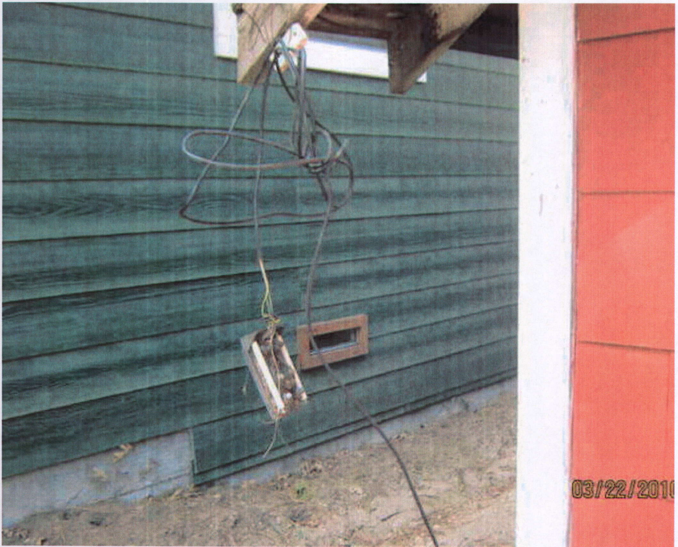
CForrey / Wires disconnected and hanging - 03/22/2010
