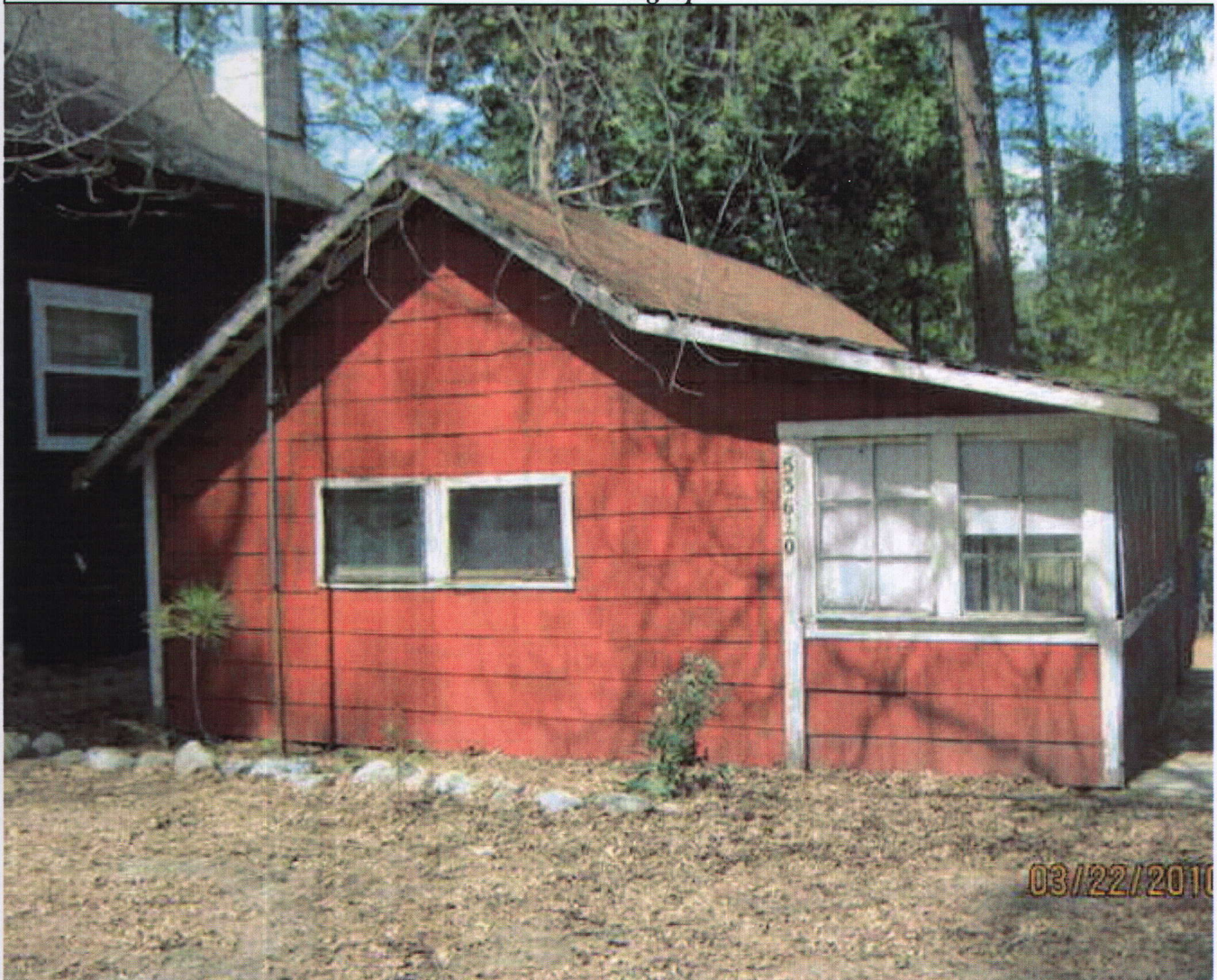
CForrey / Overview of property from street - 03/22/2010
