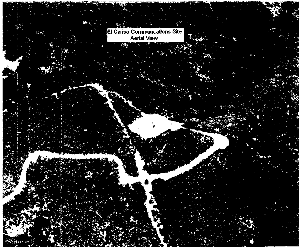
Aerial View of El Cariso Communications Site (Prior to Site Designation and Subsequent Development)
