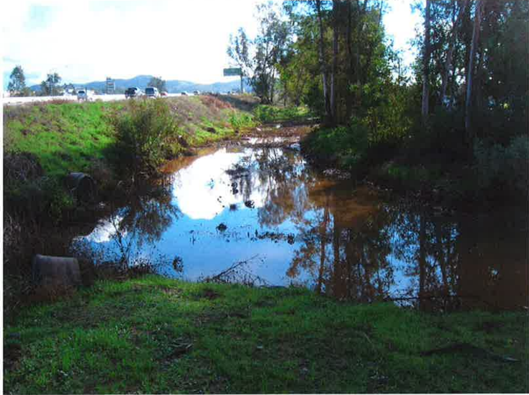
Figure 3a. View southeast, culverts on west side of I-15 Freeway, December 23, 2010
