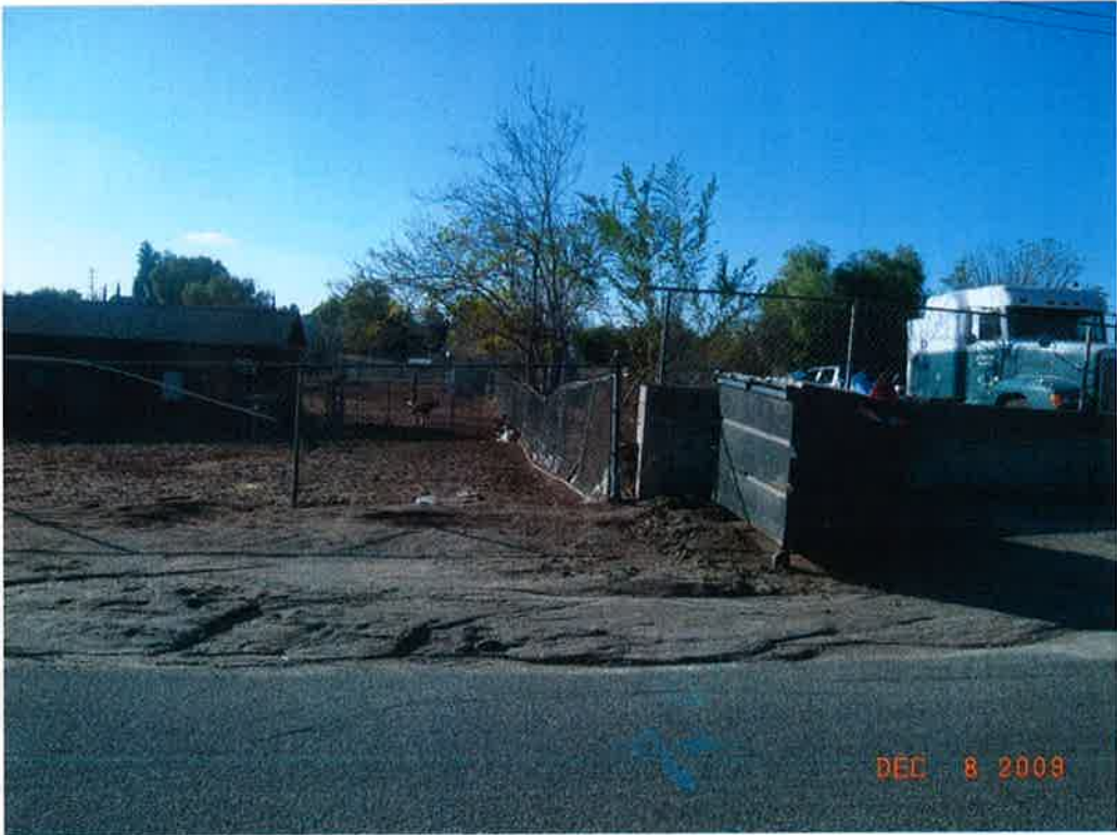
Figure 8 – Photo # 4: Beach Street, north of 55 th Street, facing west.
