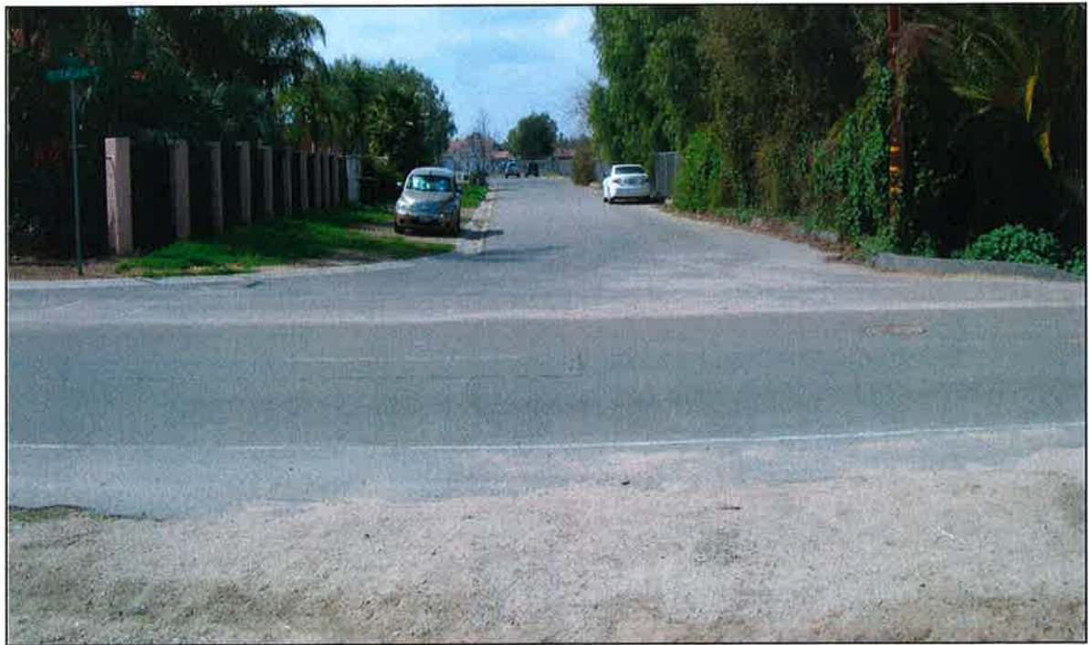
Figure 7. Norco MDP Lateral N-1D and Norco - Spirit Knoll Court Storm Drain. Intersection of Spirit Knoll Court and Temescal Avenue, Spirit Knoll Court looking west.
