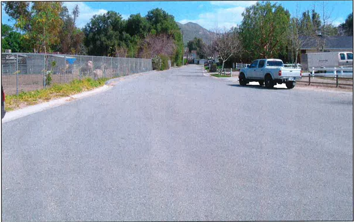
Figure 8: Norco MDP Lateral N-1D and Norco - Spirit Knoll Court Storm Drain. Spirit Knoll Court looking east.
