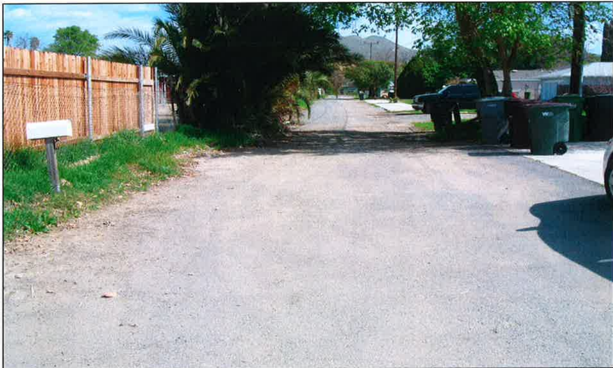
Figure 11. Norco MDP Lateral N-1D and Norco - Spirit Knoll Court Storm Drain. Rose Court looking east.
