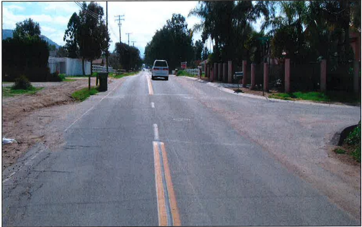
Figure 6. Norco MDP Lateral N-1D and Norco - Spirit Knoll Court Storm Drain. Intersection of Temescal Avenue and Spirit Knoll Court, Temescal Avenue looking South.
