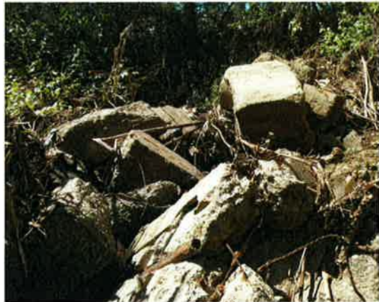
Debris dam and associated trash
