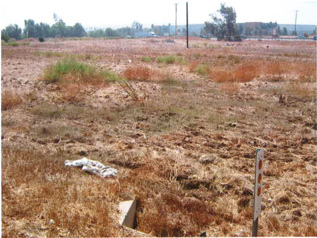
Figure 6 – Photo #3: Outlet of existing facility. Facing southwest overlooking Interstate Freeway 215.
