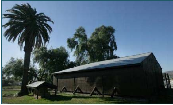
Structure built to preserve the Trujillo Adobe
