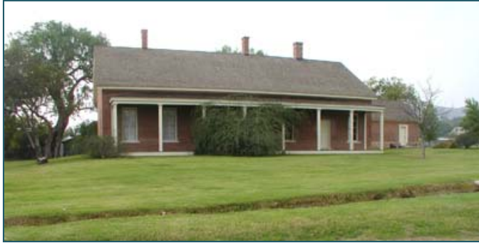
Façade of the Jensen Home
