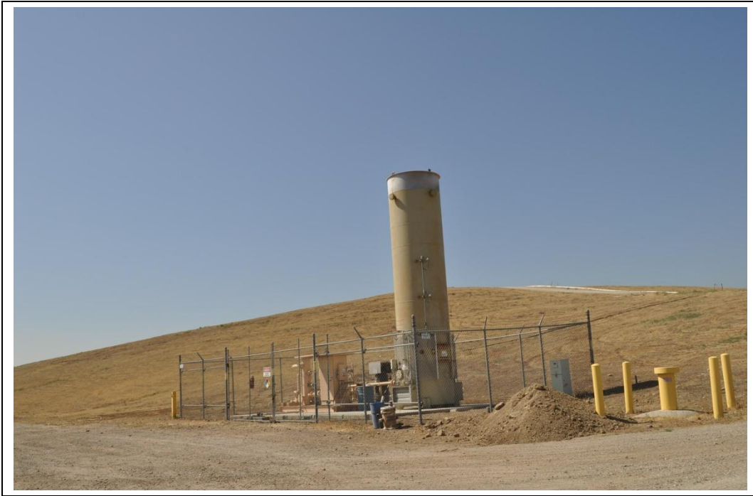
Corona entrance looking south at landfill
