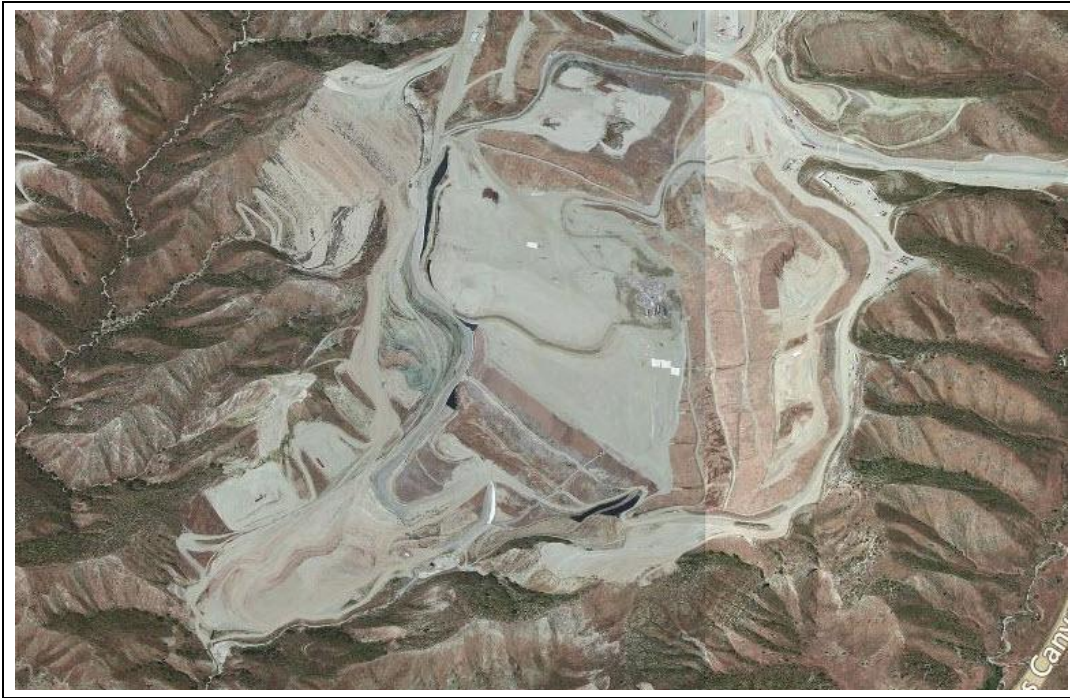
Lamb Canyon birdseye view looking north
