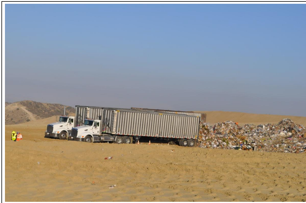
Lamb Canyon active waste drop-off area
