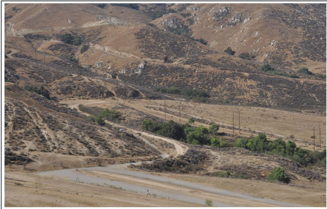
Highgrove access road
