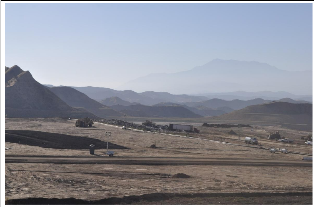
Badlands waste tipping
