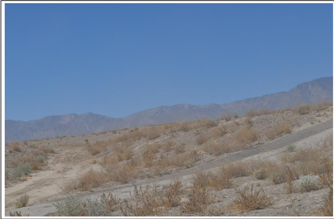
Mecca I drainage and access road to top of landfill
