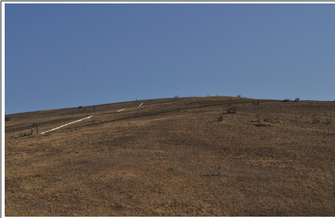
Highgrove landfill containment slope
