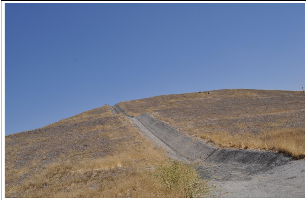
Mead Valley drainage
