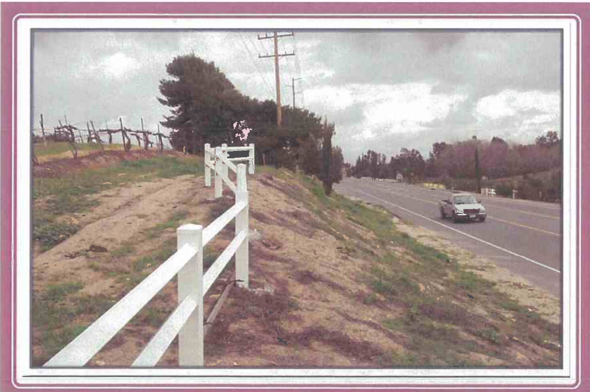
20 Condition #2 – Slope Up on N. Side
