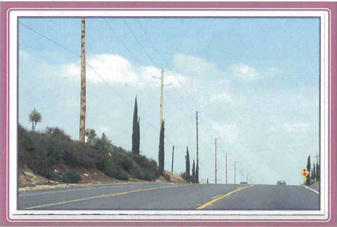
22 Condition 3 – No trail on Northwest Side of Rancho Calif. Rd. – Landscaping Only
