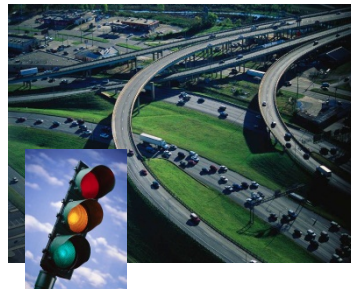
State Route 60 and Valley Way ramp and signals
