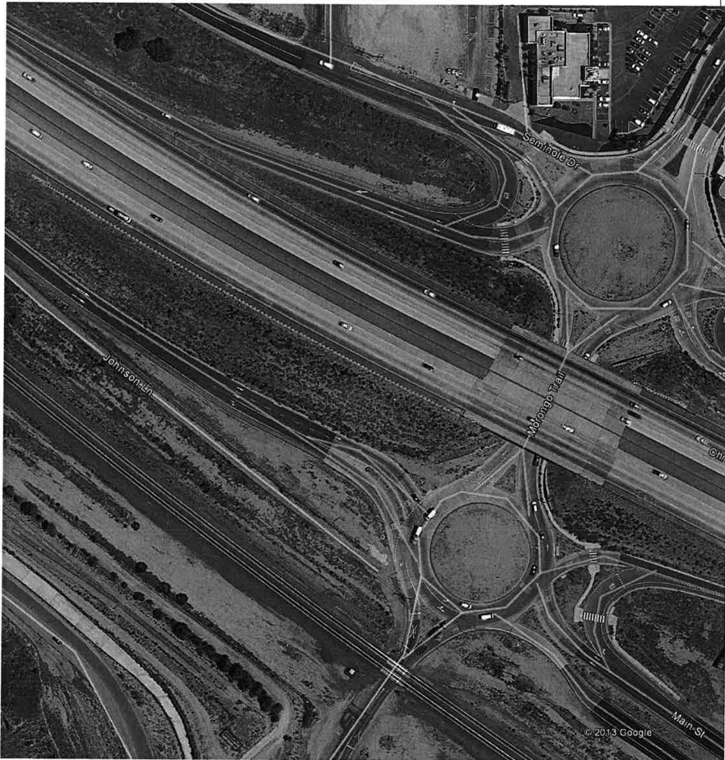
Roundabout locations - Interstate 10 at Morongo Trail
