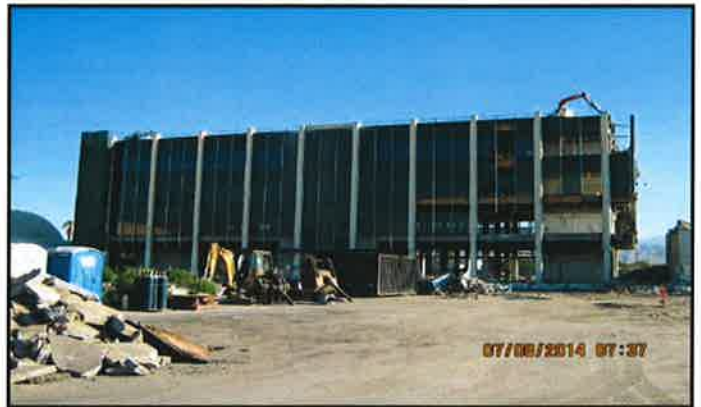
Figure 10. July 08, 2014: Demolition Equipment placed at CAC Roof
