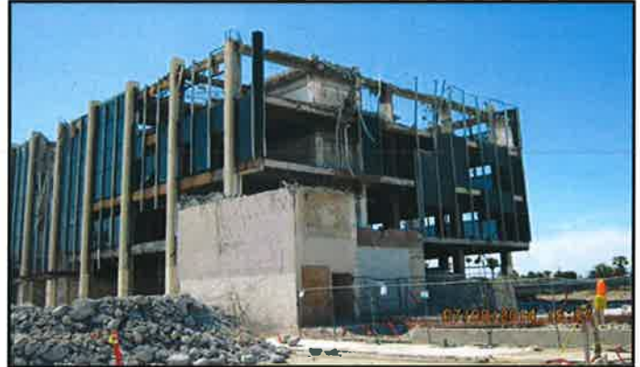
Figure 8. July 08, 2014: Demolished Roof at CAC Building
