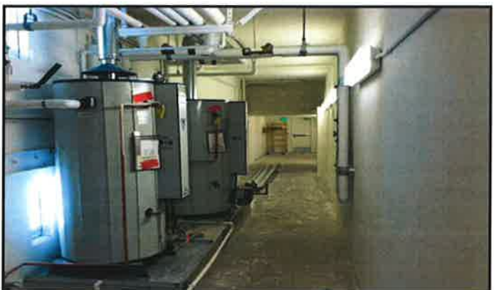
Figure 6. July 09, 2014: Completed New Mechanical Room
