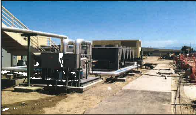
Figure 7. July 09, 2014: Completed New Existing Jail Utilities
