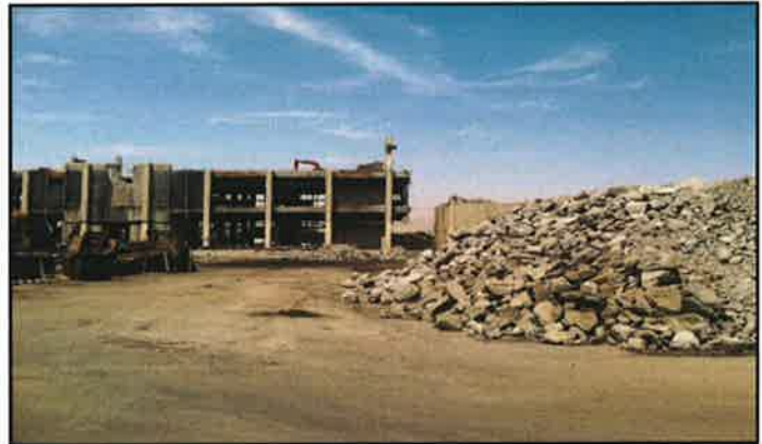
Figure 6. August 01, 2014: North View, Late July
