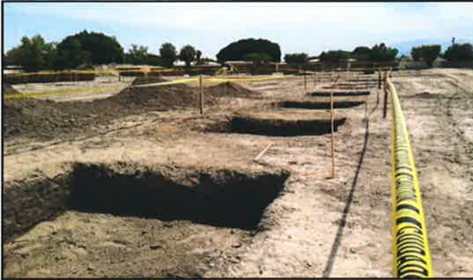
Figure 7. August 01, 2014: Spread Footing Foundation
