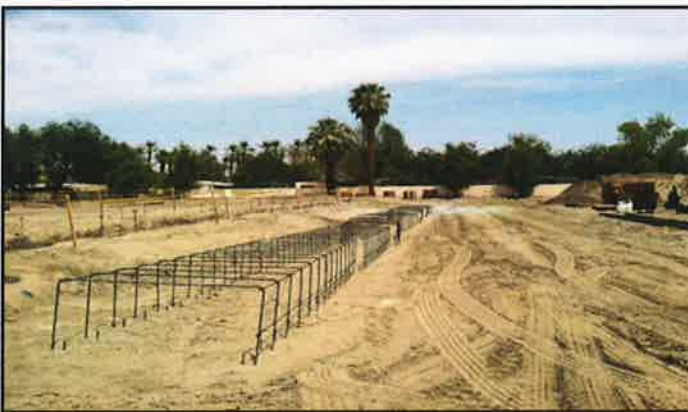
Figure 9. August 01, 2014: Foundation (Grade Beam) Steel Reinforcement
