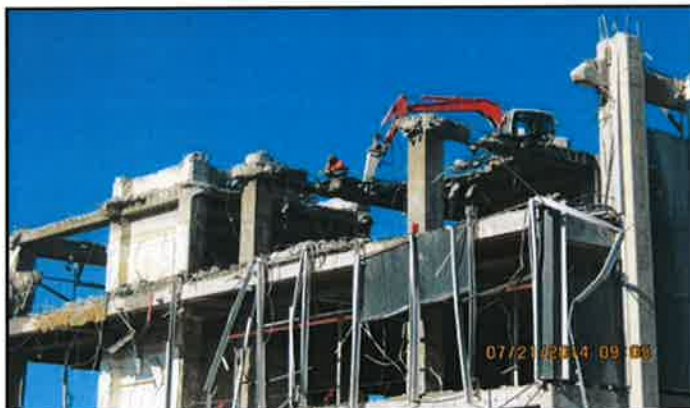
Figure 5. July 21, 2014: Demolition Crew and Equipment at Third Floor
