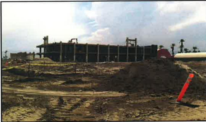
Figure 7. August 01, 2014: Southwest View, Late July
