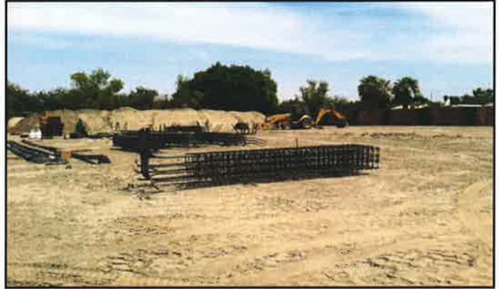
Figure 8. August 01, 2014: Ground Level Steel Reinforcement
