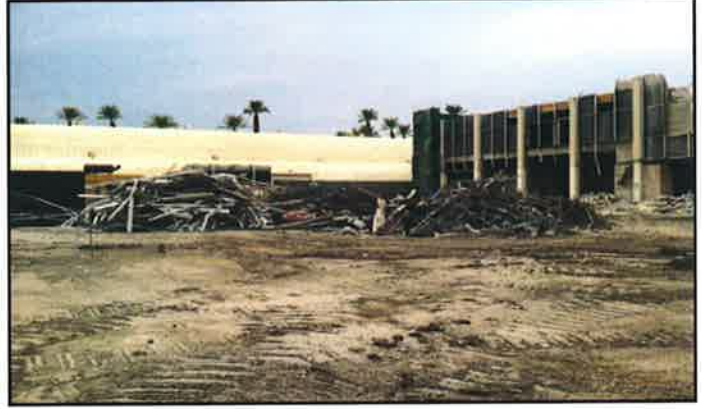
Figure 8. August 01, 2014: Steel and Metal Demolition Debris
