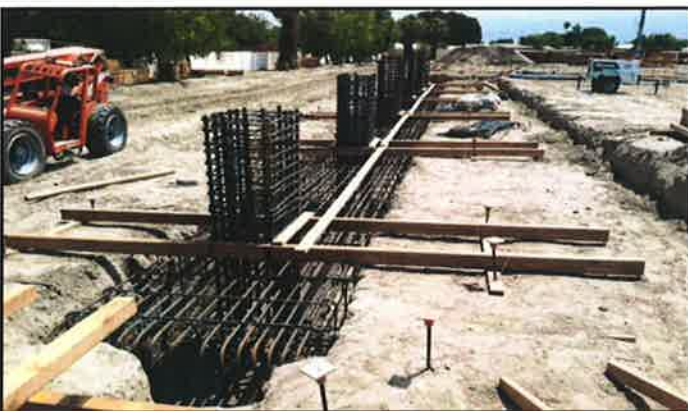
Figure 11. August 01, 2014: Reinforced Grade Beam with Column Reinforcement
