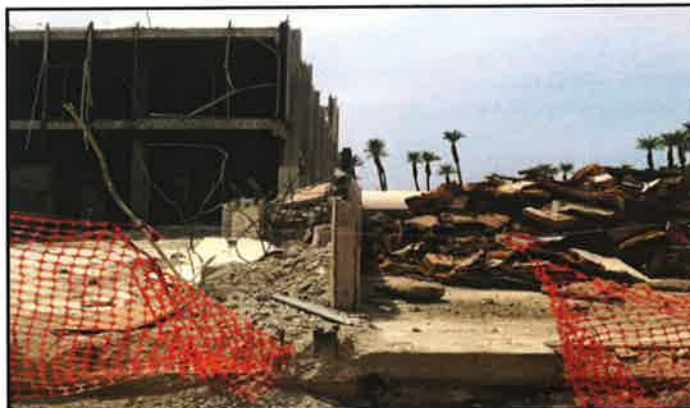
Figure 11. August 01, 2014: View North at CAC Building Demolition
