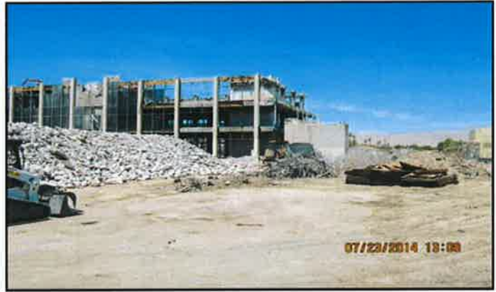
Figure 4. July 23, 2014: Demolition of the Third Floor, CAC Building, Northwest View
