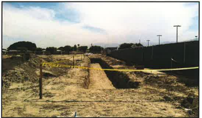
Figure 6. August 01, 2014: Grade Beam Foundation
