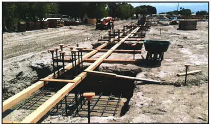
Figure 10. August 01, 2014: Spread Footings with Column Reinforcement
