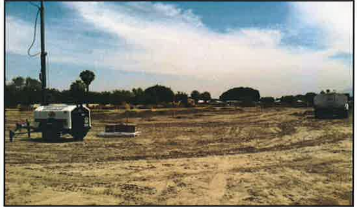
Figure 2. August 01, 2014: South East View
