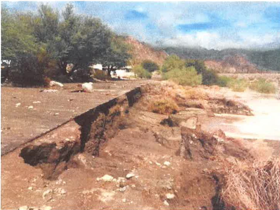
Erosion on banks of the road
