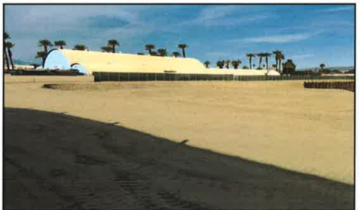
Figure 12. January 08, 2015: View from South, Northwest
