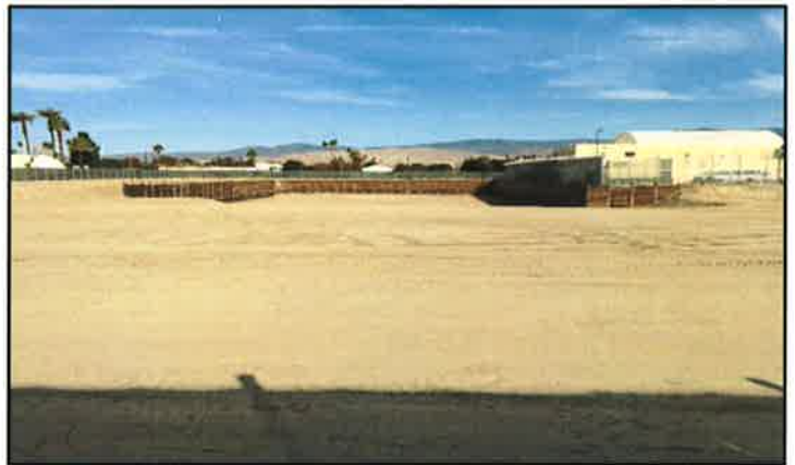
Figure 10. January 08, 2015: View from South, North to Excavation
