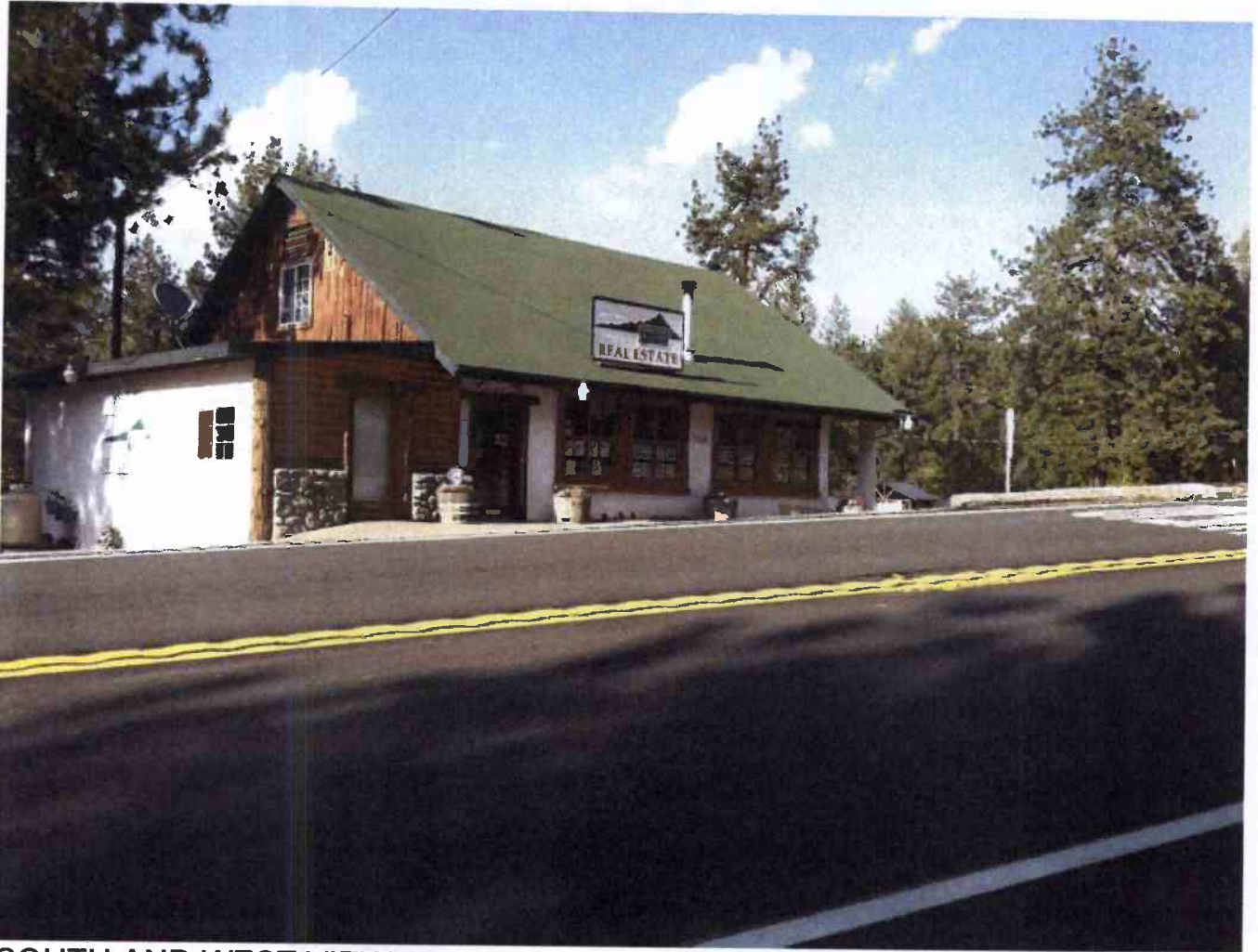
SOUTH AND WEST VIEW
