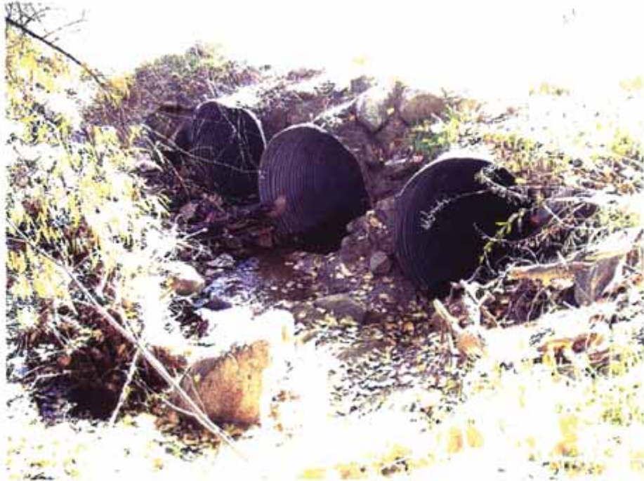
Figure 1-2 – Warm Springs – Looking downstream at Los Alamos Road Culvert
