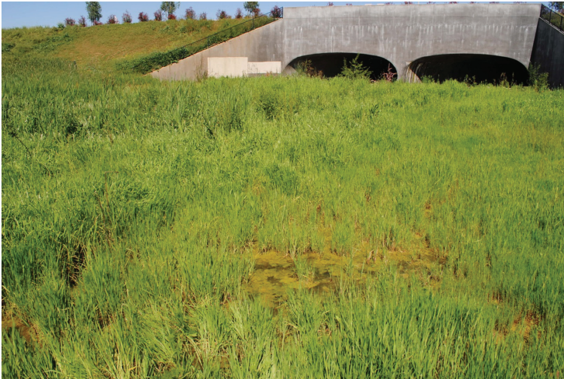
Photograph 4: Another view of HydroArch Culvert Under Leon Road - facing north
