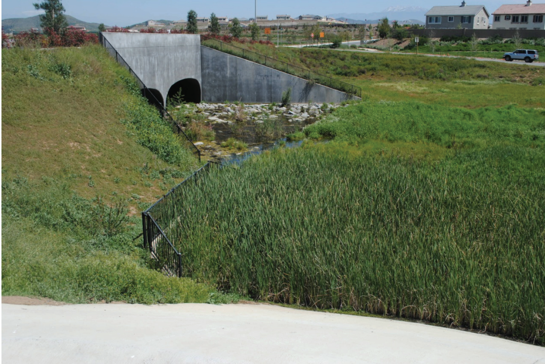
Photograph 3: HydroArch Culvert Under Leon Road – facing east towards Briggs Road
