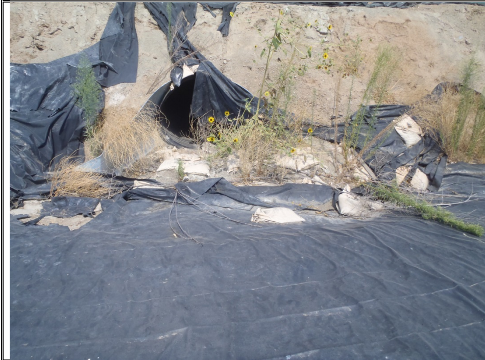
Photo 50 Date: 09-09-2013 Feature: Drainage 11 Direction: Northwest Description: Downstream view of Drainage 11.
