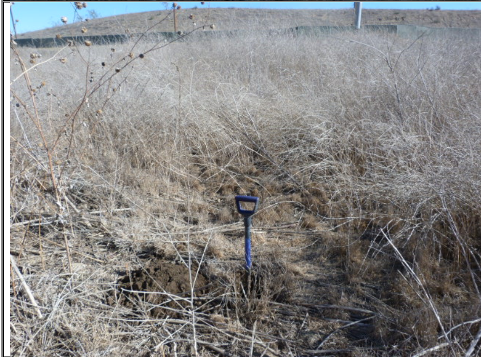
Photo 82 Date: 01-16-2014 Feature: Drainage 16- French Valley Creek Direction: East Description: Photo of SP-57.
