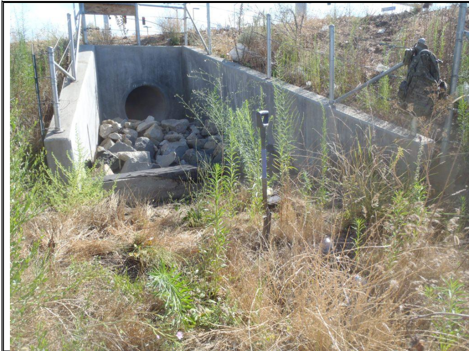
Photo 43 Date: 08-20-2013 Feature: Drainage 9 Direction: South Description: Upstream view of SP-24.
