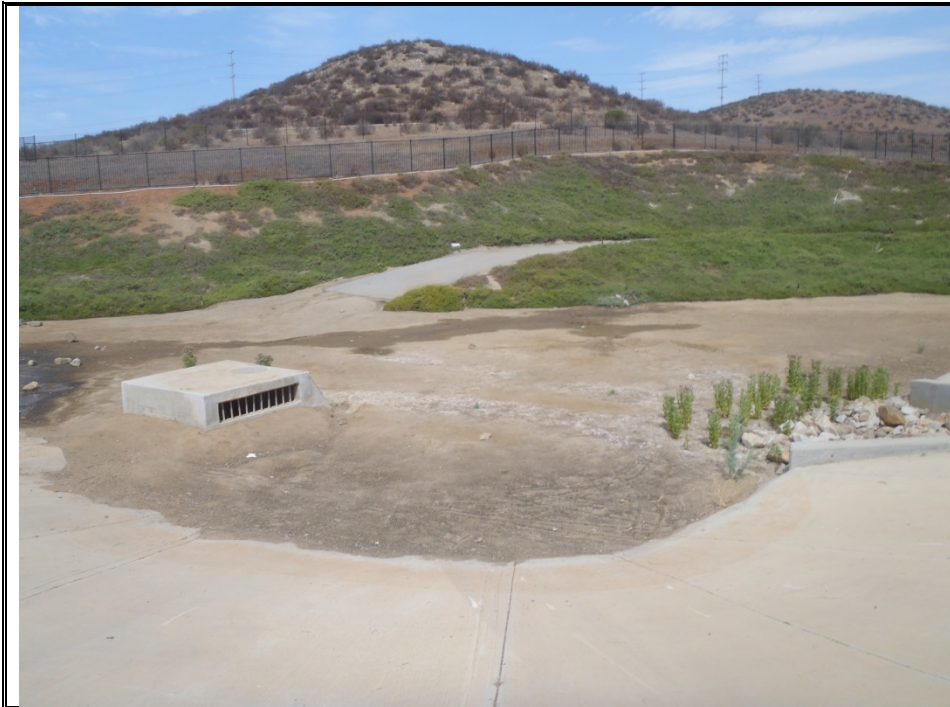
Photo 49 Date: 09-09-2013 Feature: Basin 1 Direction: North Description: Overview of Basin 1.
