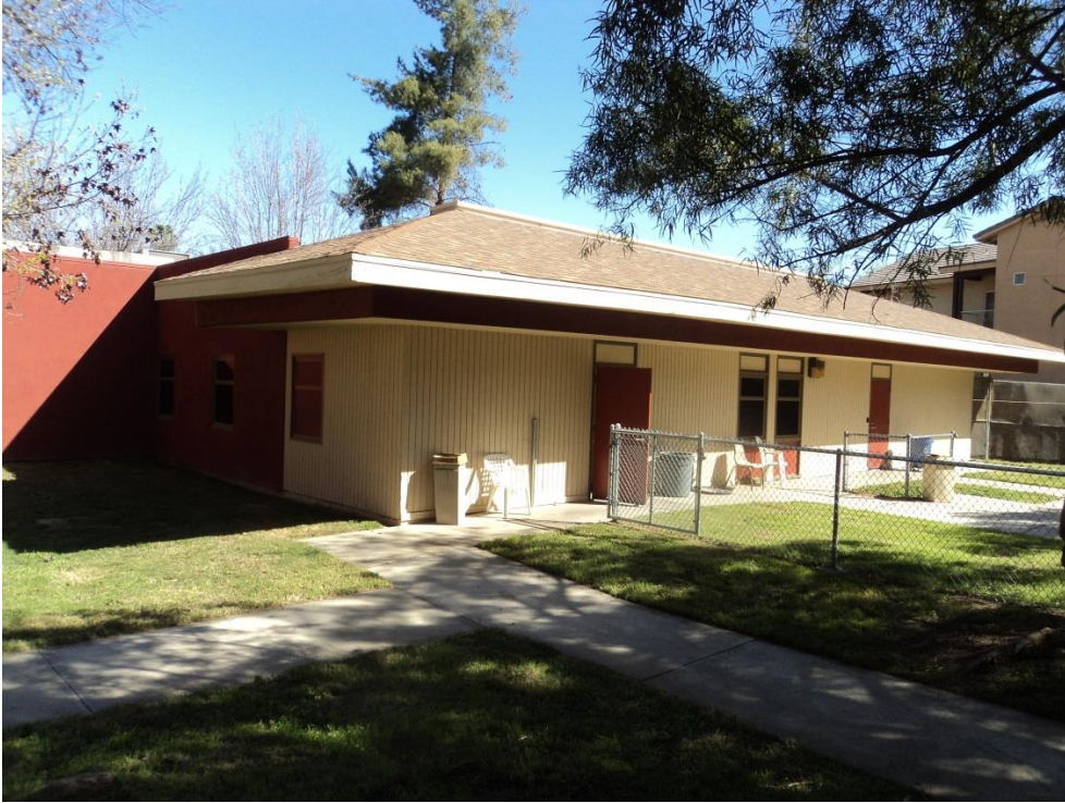
Photograph 1- Illustrates ACM transite panels below windows in Building A.
