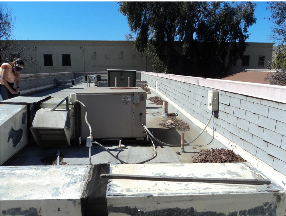
Photograph 2 - Illustrates the roof and roof penetrations on building C.
