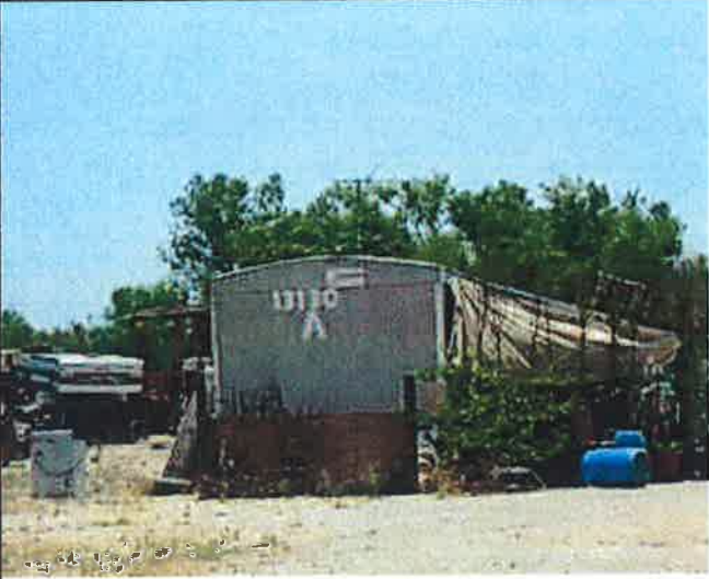
Rubbish and excessive outside storage-JMorri 6/24/14
