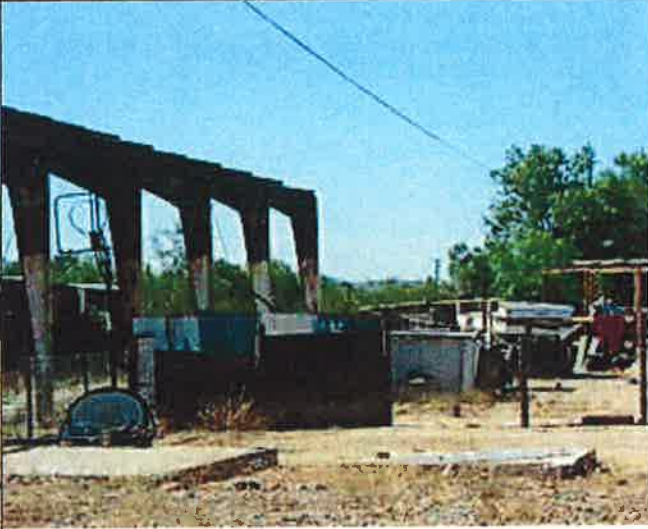
Rubbish and excessive outside storage remains JMorris 8/5/14
