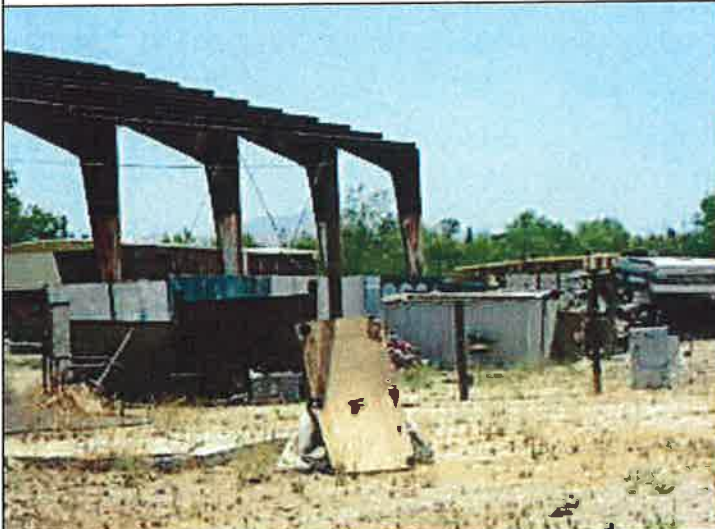
Rubbish and excessive outside storage-JMorris 6/24/14
