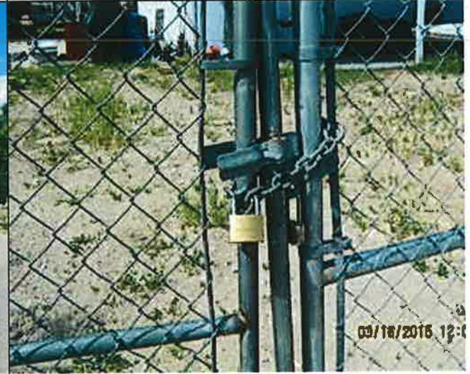
Photo taken from the right of way D Jurden, CET
