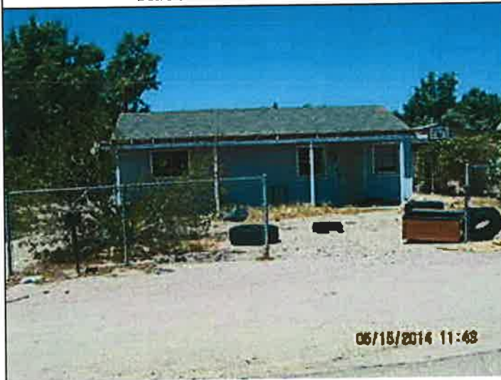
Photo taken from the right of way D Jurden, CET
