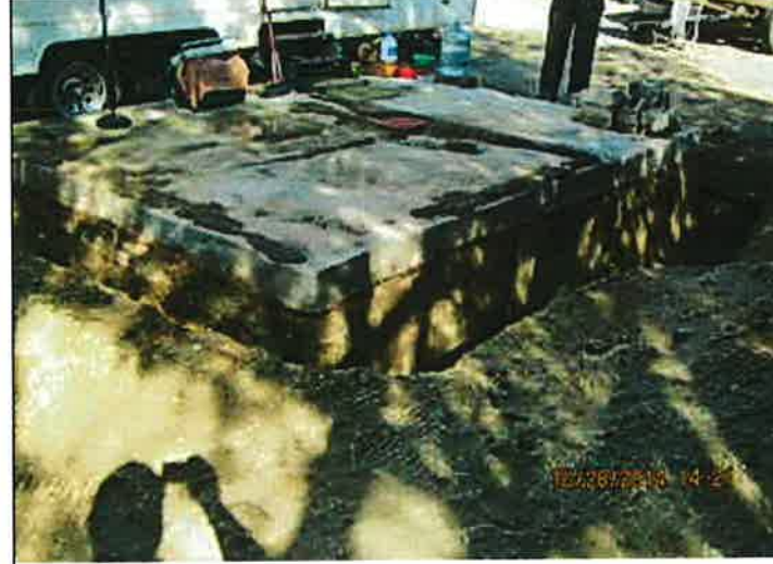
E. Torres; squatter excavating around septic
