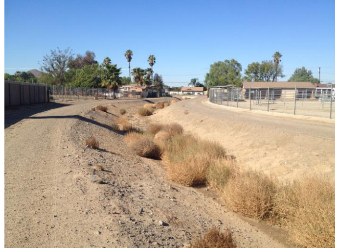
Location 3: Inlet 1 facing west, downstream.
