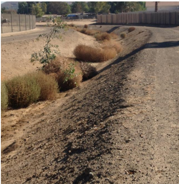
Location 4: Facing east, upstream.
