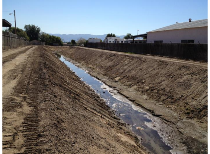
Location 16: Flowing Water – facing south, downstream. Standing water is from inlet conveying nuisance flows into the channel.
