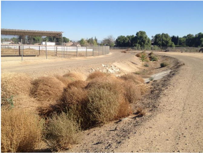
Location 3: Inlet 1 facing northeast, upstream.
