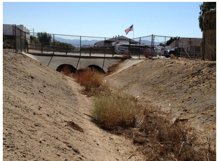
Location 15: North of Sixth Street – facing south, downstream towards Sixth Street.
