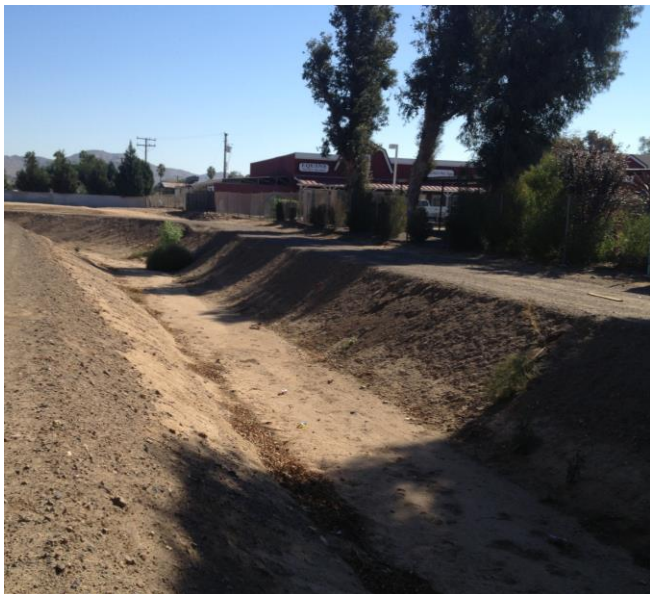
Location 11: Facing east, upstream.
