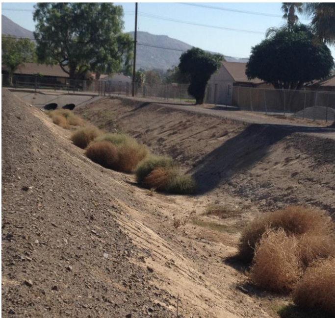
Location 6: Facing east, upstream towards Corona Avenue.
