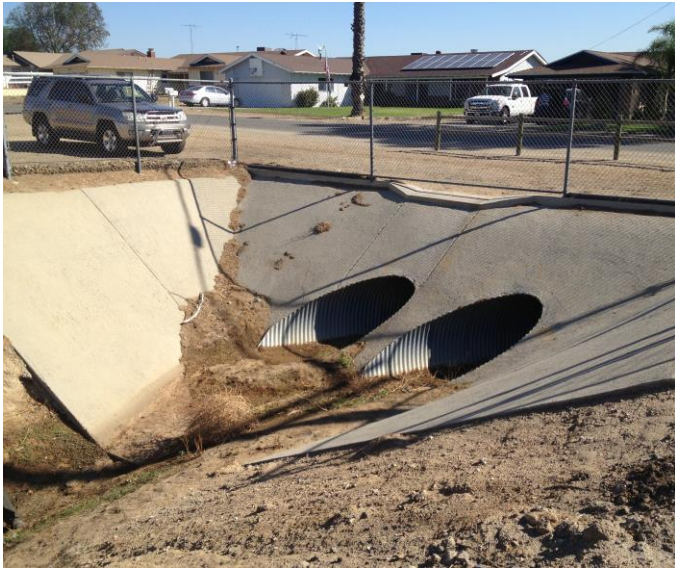
Location 5: Facing east, upstream towards Corona Avenue.
