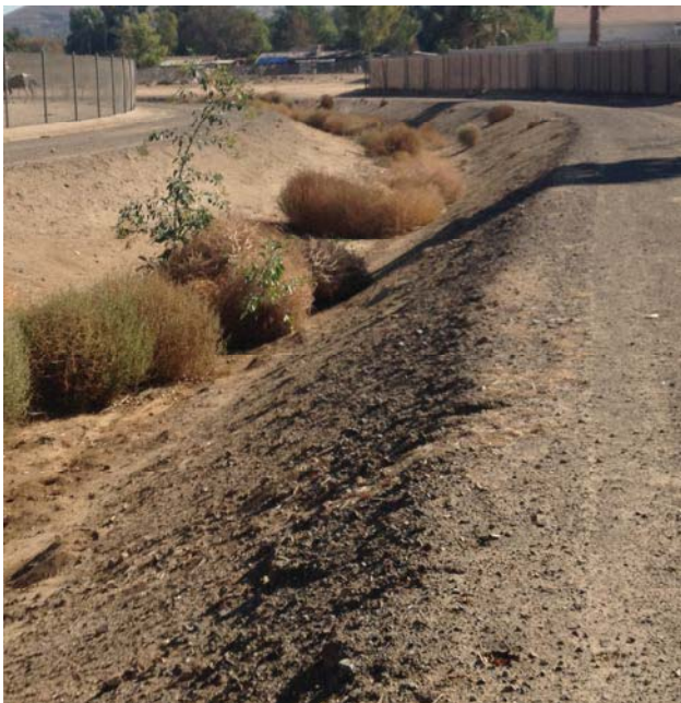
Location 4: Facing east, upstream. Bed 6ft. Bank 27ft.
