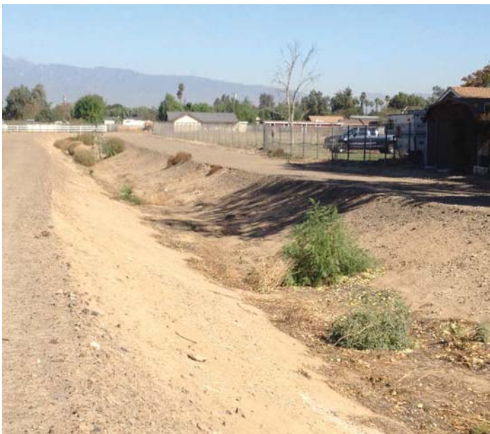
Location 8: Facing north, upstream. Bed 7ft. Bank 30ft.
