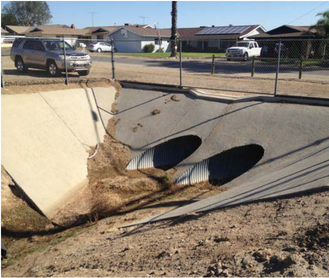
Location 5: Facing east, upstream towards Corona Avenue. Bed 5ft. Bank 40ft.
