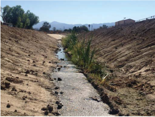
Location 21: Facing south, downstream. Bed 13ft. Bank 37ft. Wetland vegetation along toe of slope.
