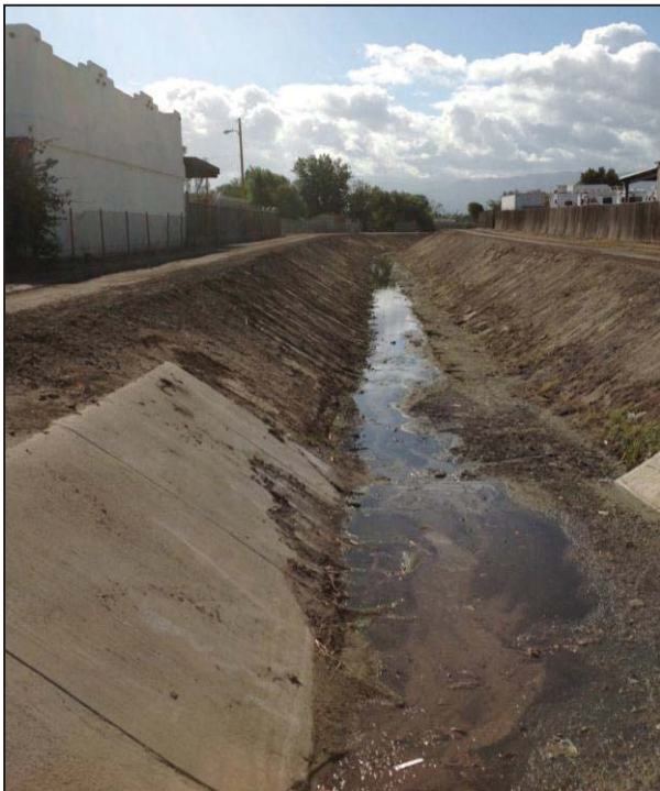
Figure 7. Channel, view south from 6 th Street
