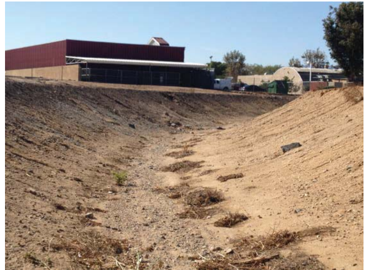
Location 9: Facing southwest, downstream. Bed 5ft. Bank 34ft.
