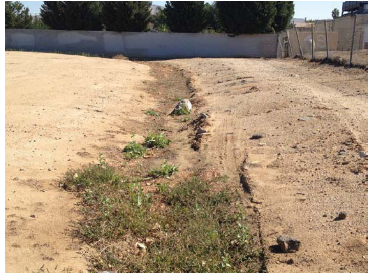
Location 12: Swale facing east, upstream. Partially vegetated area with Mexican sprangletop.
