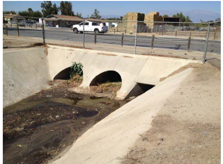
Location 19: Flowing Water – facing north, upstream towards Sixth Street.
