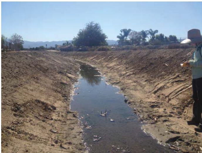
Location 20: Facing southwest, downstream. Bed 9ft. Bank 26ft. Evidence of recent maintenance activities (scrape marks along channel slopes)
