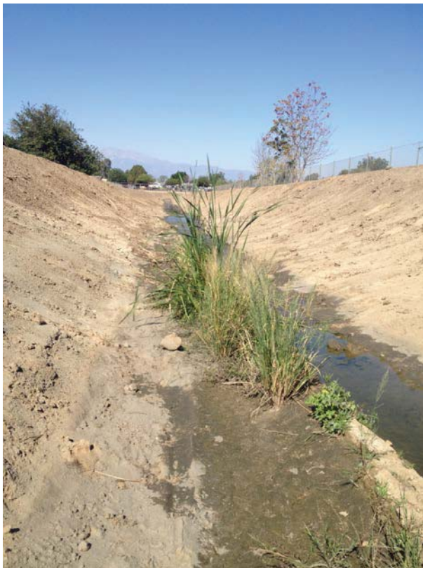
Sample Point 2: Overview photograph facing north, upstream.
