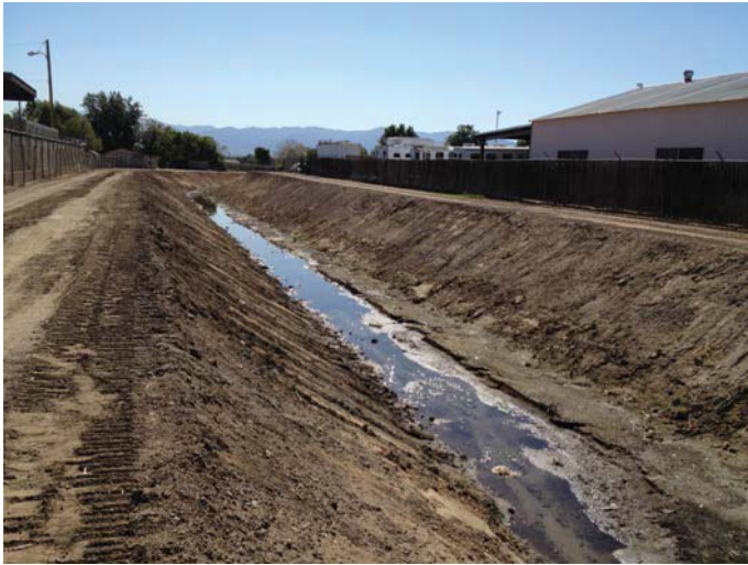
Location 19: Flowing Water – facing south, downstream. Standing water is from inlet conveying nuisance flows into the channel.
