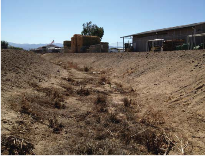
Location 17: Facing southwest, downstream towards Sixth Street. Bed 8ft. Bank 28ft.
