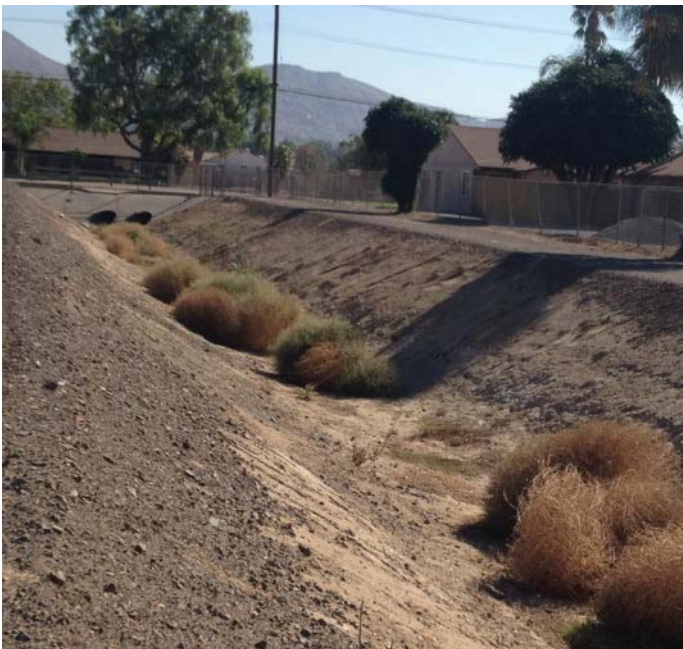
Location 6: Facing east, upstream towards Corona Avenue. Bed 7ft. Bank 36ft.
