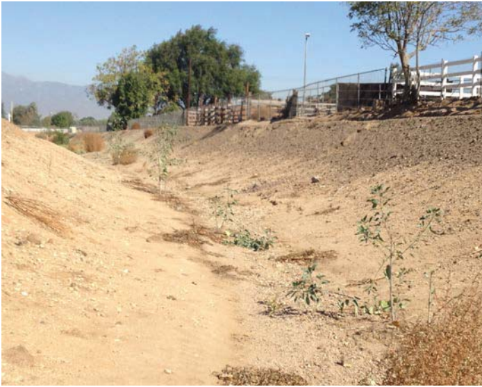
Location 9: Facing north, upstream. Bed 5ft. Bank 34ft.
