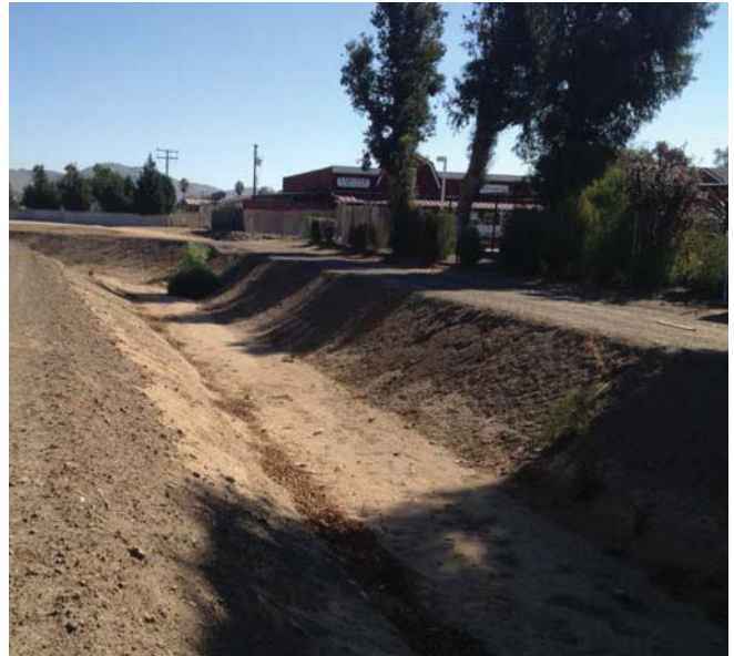
Location 14: Facing east, upstream. Bed 8ft. Bank 24ft.
