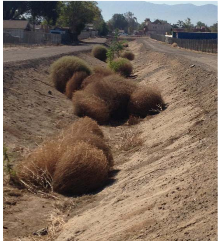
Location 7: Facing southwest, downstream. Bed 7ft. Bank 30ft.
