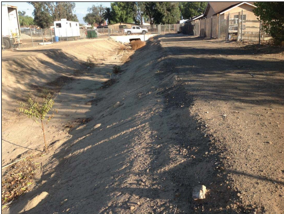
Figure 5. Channel, view north towards Rose Court
