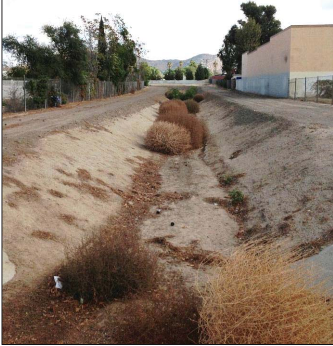
Figure 6. Channel, view east from Valley View
