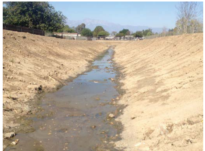
Location 21: Facing north, upstream. Bed 13ft. Bank 37ft.
