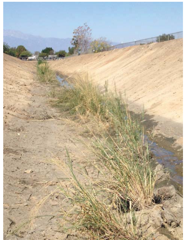
Sample Point 3: Overview photograph facing north, upstream.
