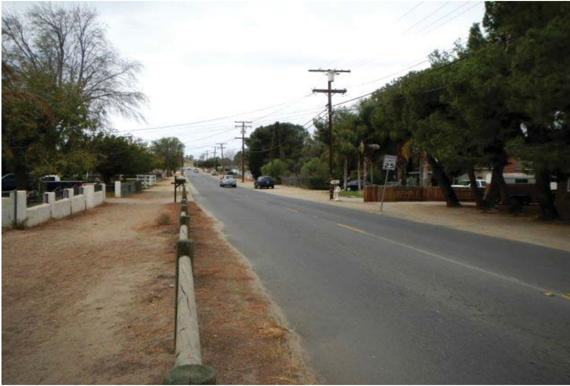
Photograph 7 - Looking west along Detroit Street. Note the pole-mounted transformer on the north side of the street.
