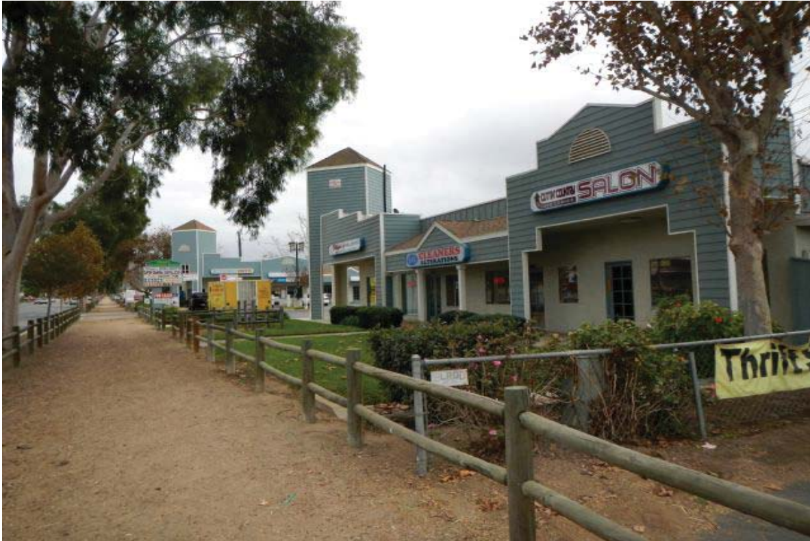
Photograph 17 - Looking east along 6th Street at a strip mall with a cleaners, restaurants, and salon.
