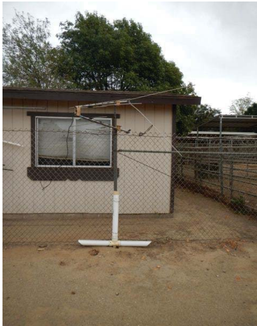
Photograph 12 - PVC "T" pipes located along the perimeter of the subject property.
