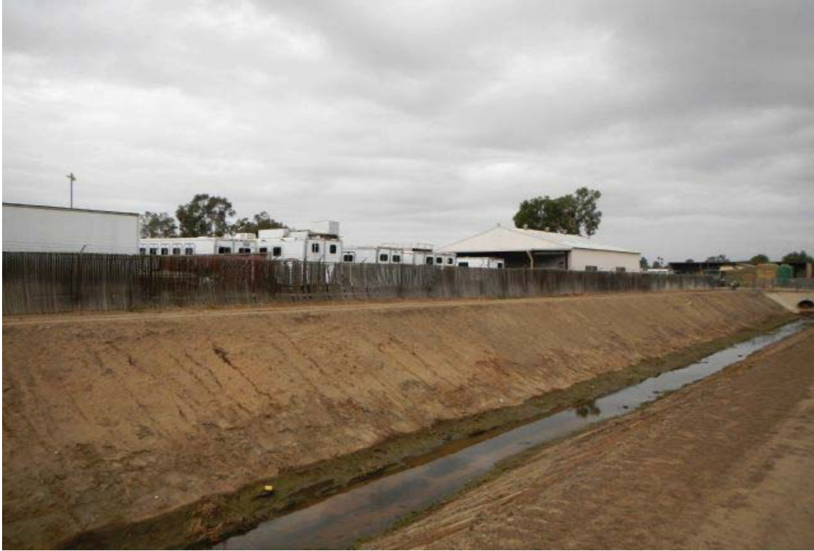
Photograph 13 - Trailer sales and service located to the west of the 6th Street crossing.
