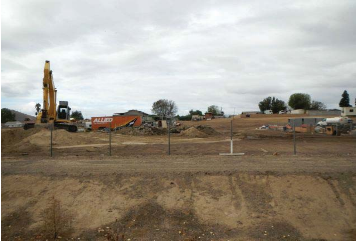
Photograph 21 - Equipment and debris storage located on an western-adjacent property at the northeast termination of the subject property.
