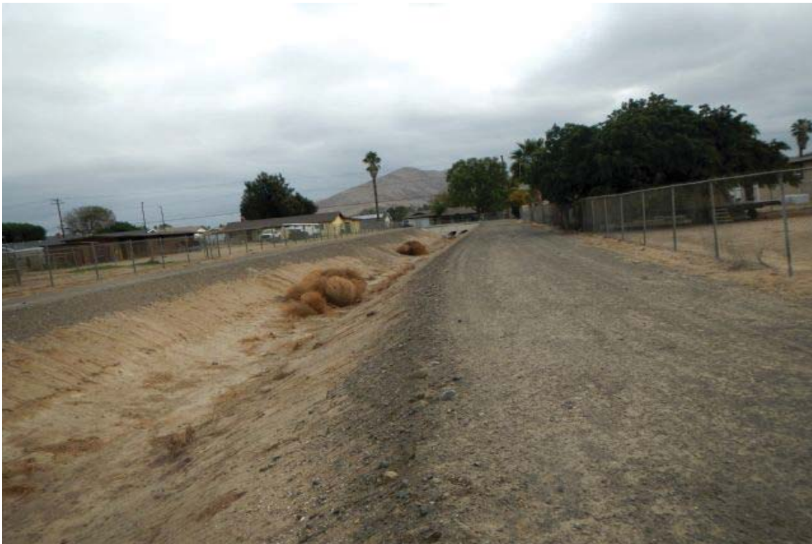
Photograph 10 - Looking east toward the Corona Avenue crossing.
