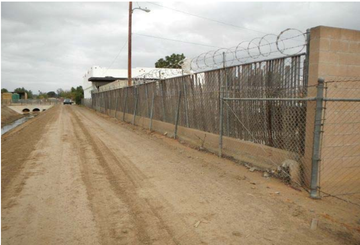
Photograph 2 - Looking north at the 6th Street bridge and culvert. A fence company is located to the east and an animal feed store is located on the north side of 6th Street.
