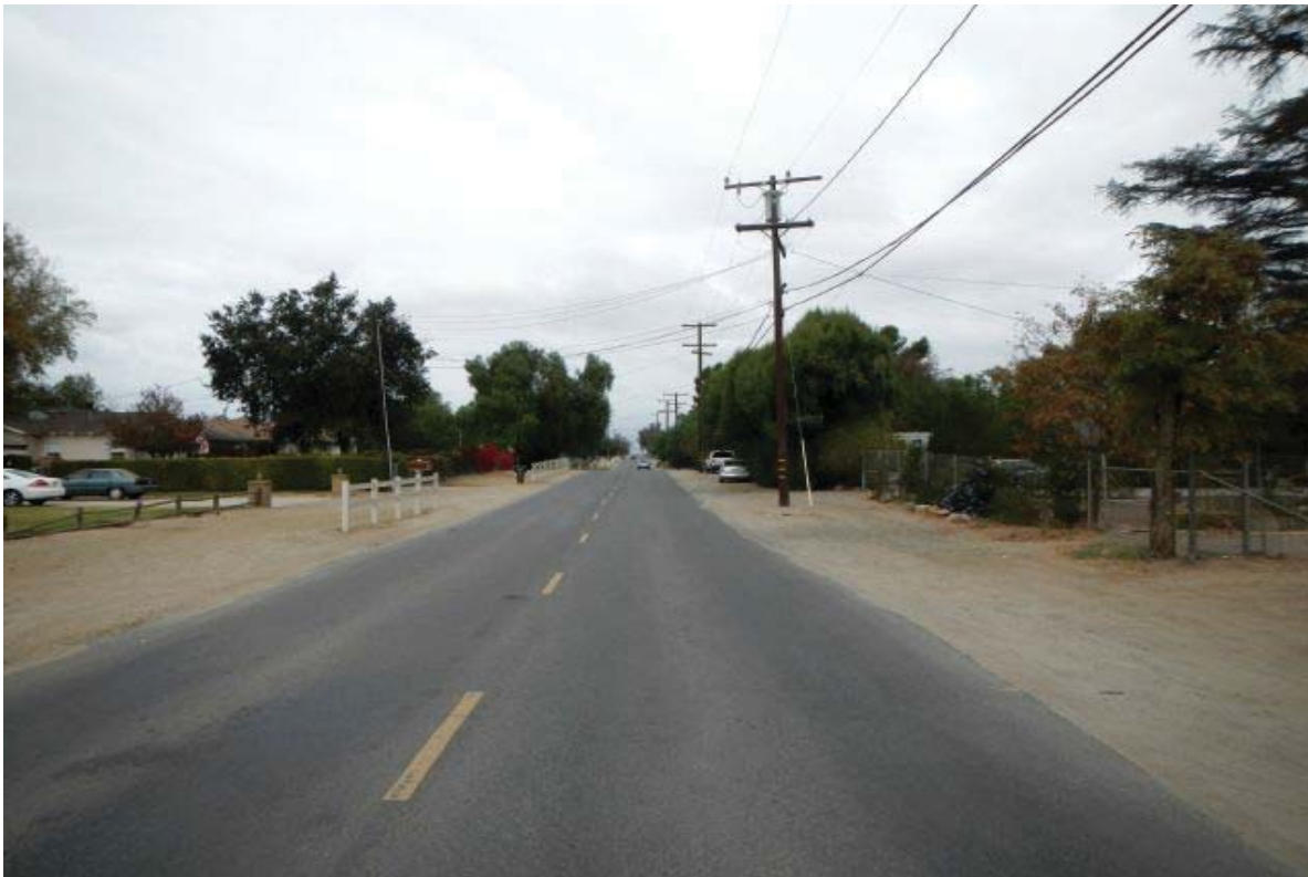
Photograph 6 - Looking north on Valley View. Note the pole- mounted transformer on the east side of Valley View Avenue.
