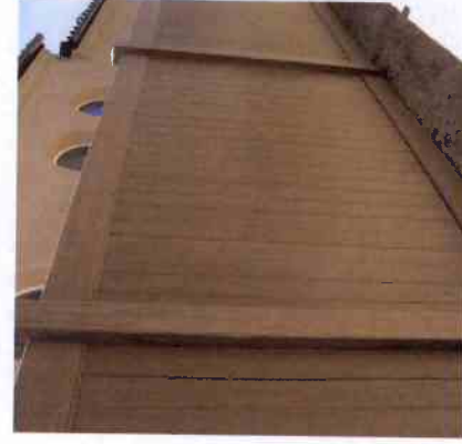
Vinyl Fencing Example
