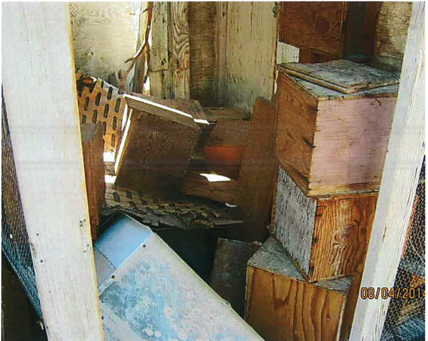
Inside str. # 4. Scrap wood throughout. 17 of 20. RH - 08/04/2014
