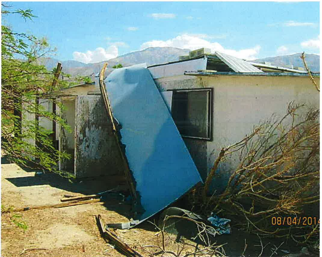
Structure # 3. Roof piece in front of entrance. 11 of 20. RH - 08/04/2014
