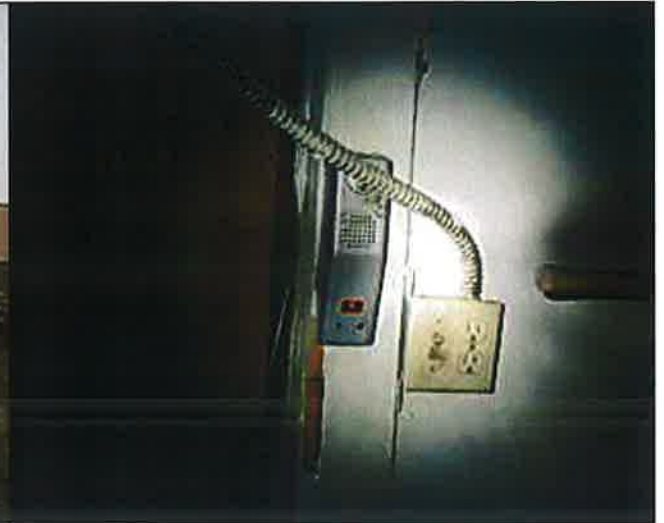
-09/26/14 - Initial Inspection SSST Verified - NC 6,15 - Pike
