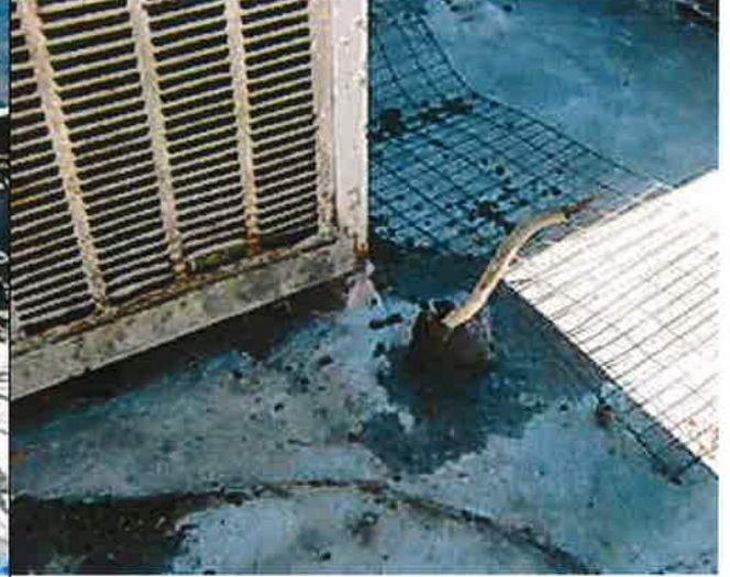
09/26/14 - Initial Inspection SSST Verified - NO 6,15 - Pike
