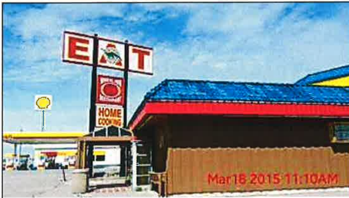
E. Torres; substandard structure continues to deteriorate
