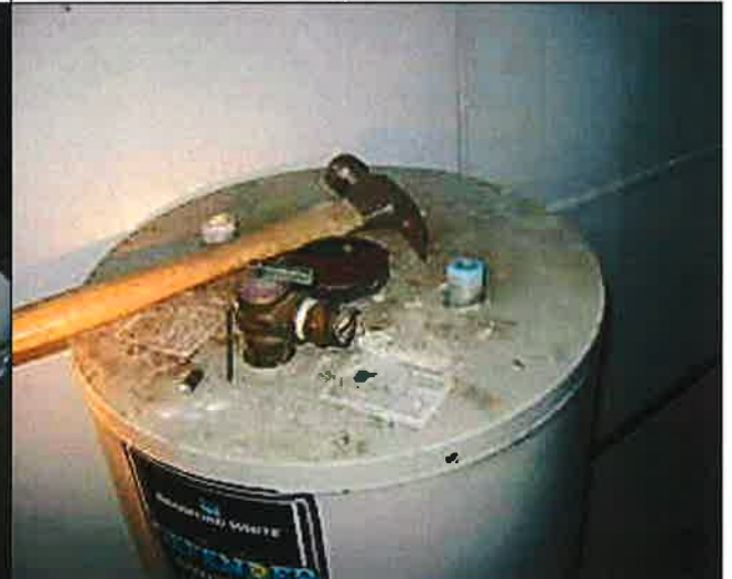
09/26/14 - Initial Inspection SSST Verified - NO 1,2 - Pike
