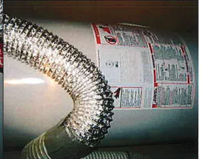
09/26/14 - Initial Inspection SSST Verified - NO 1,2,4 - Pike
