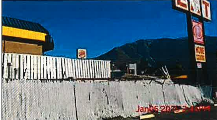
E. Torres; structure remains in substandard condition
