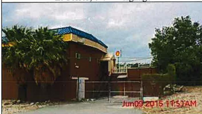
E. Torres; additional broken or missing windows
