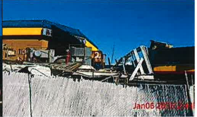
-E. Torres; structure remains in substandard condition
