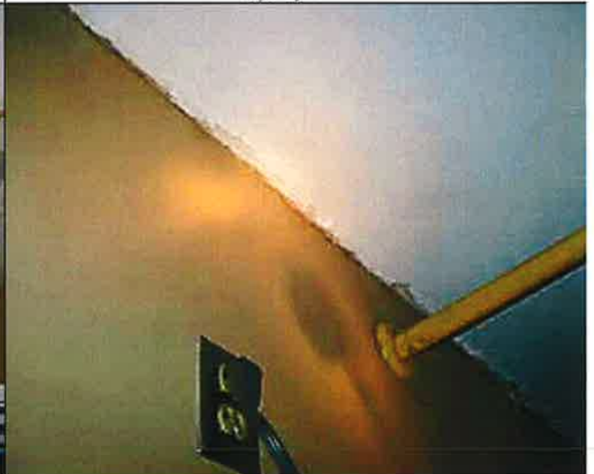
09/26/14 - Initial Inspection SSST Verified - NO 11 - Pike
