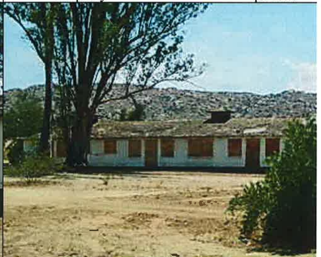
Property remains in violation. Lpadilla
