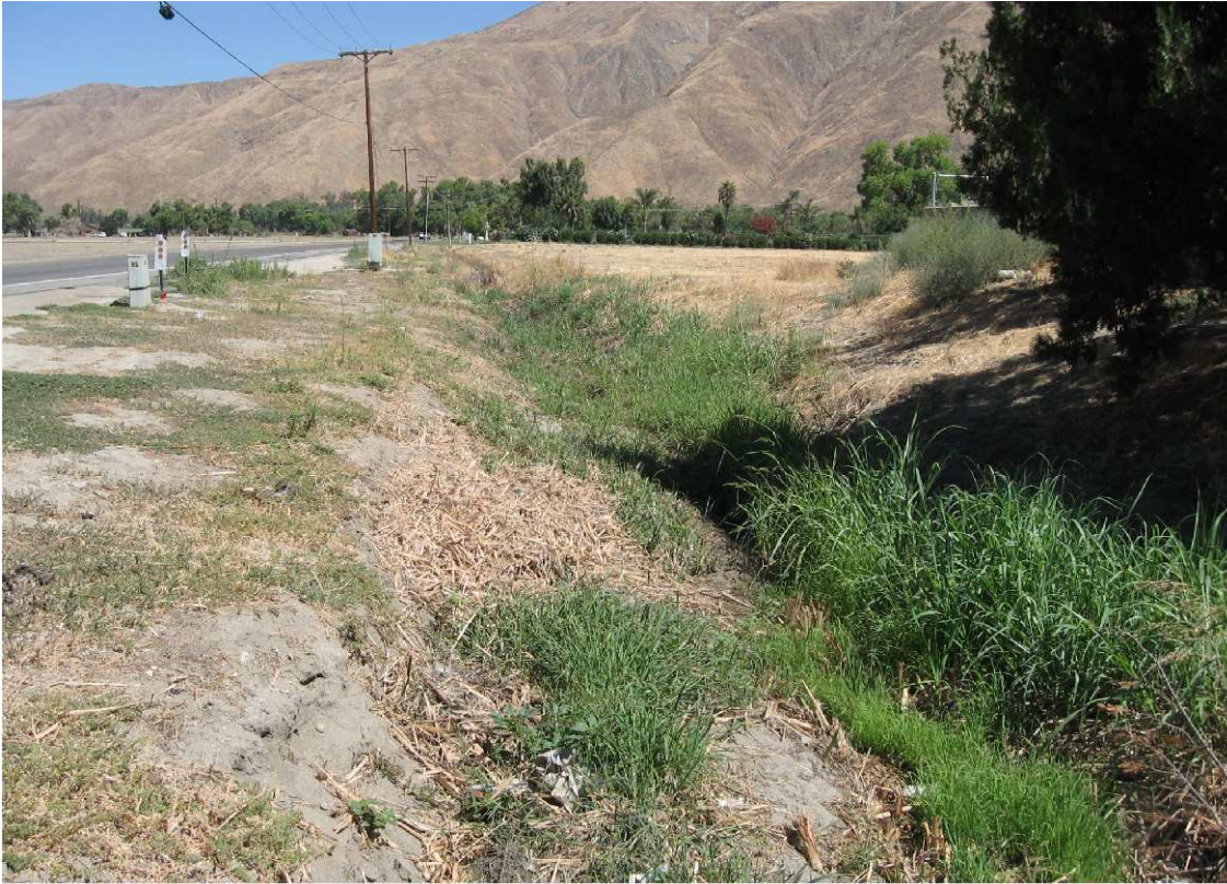
Photograph 1: View of survey area for Line H looking North. Photo depicts typical road side swale parallel to State Street.
