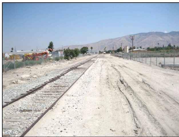
Figure 6. A segment of the San Jacinto Valley Railway within the APE (view to the north, photo taken on July 18, 2008).
