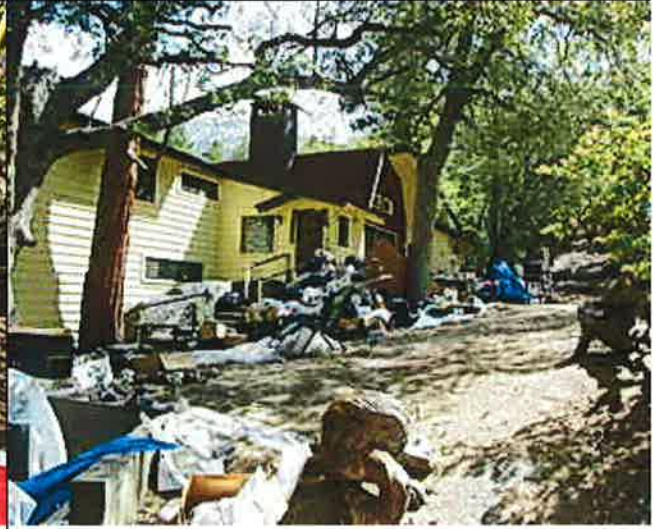
the violation remains with deplorable condition
