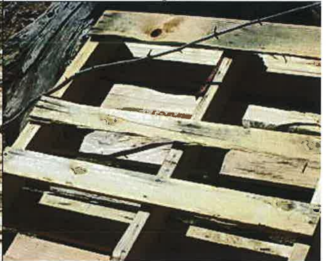
current photo of site
