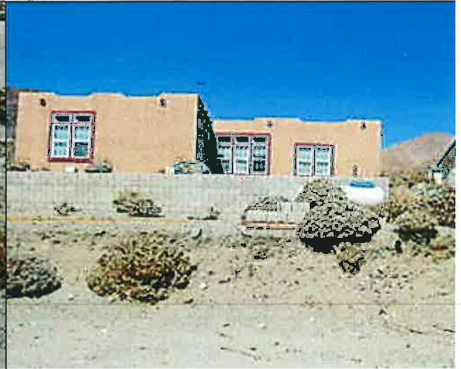
09/28/12 - Accumulated Rubbish - Pike
