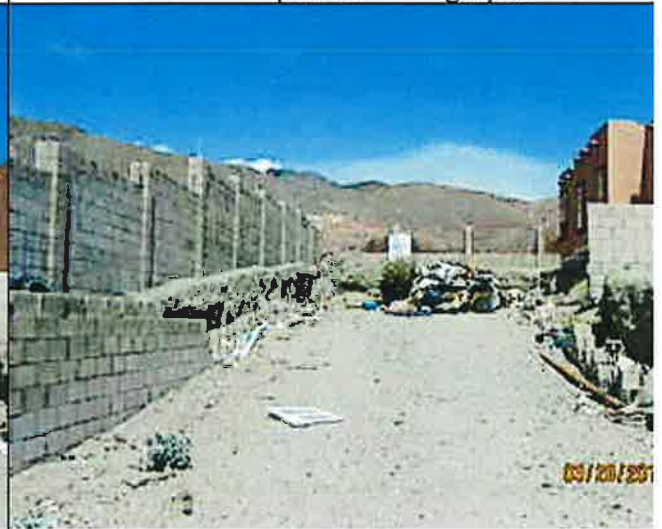
Accumulated rubbish remains. J Chamberlain
