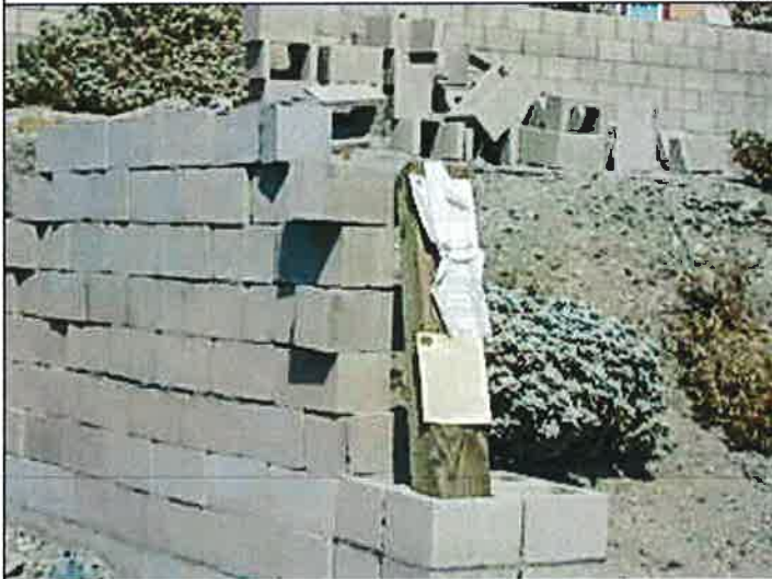
09/28/12 - Accumulated Rubbish - Pike
