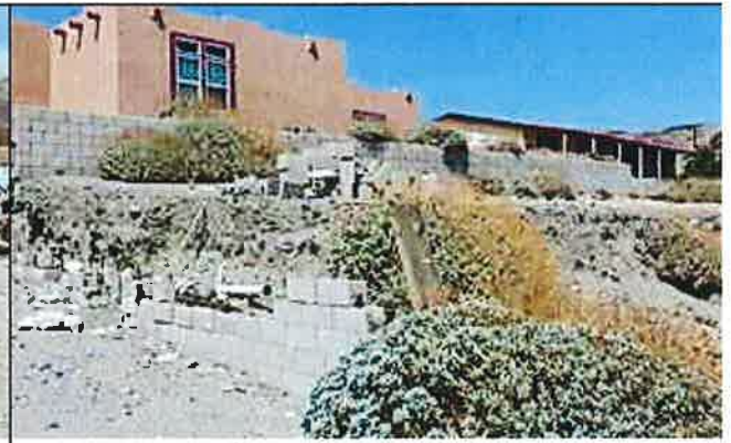
Unpermitted Grading/Cut 5/7/15 J. Cole
