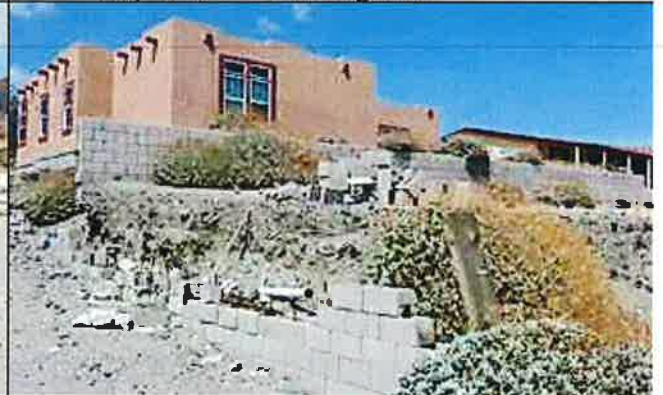
Unpermitted Grading/Cut 5/7/15 J. Cole
