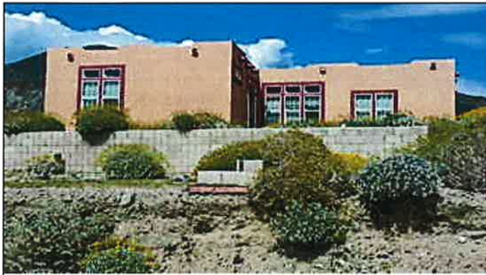
Unpermitted Grading/Cut 3/18/15 J. Cole
