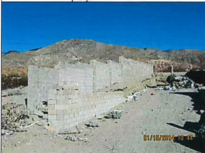
Unpermitted Grading 1/15/14 J. Cole
