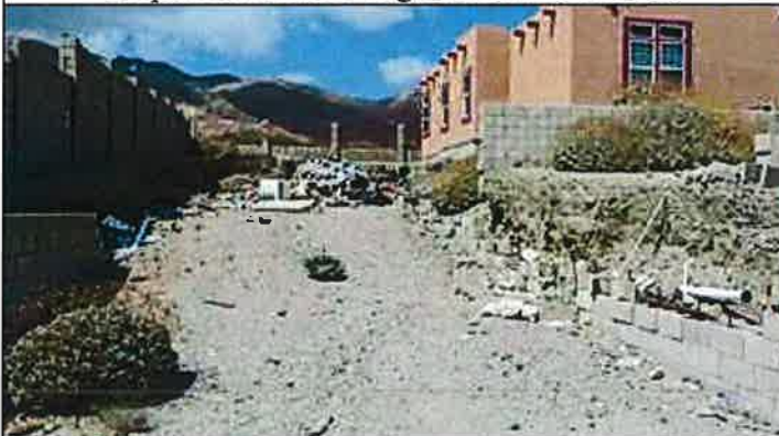
Unpermitted Grading/Cut 5/7/15 J. Cole
