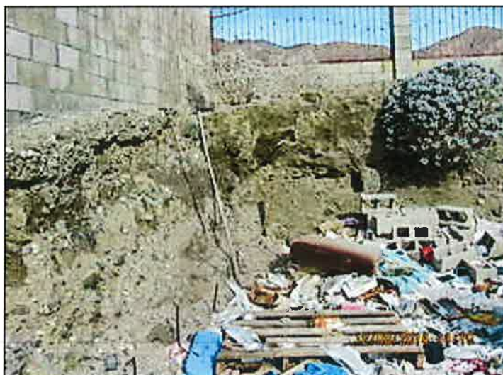
Unpermitted Grading/Cut 12/8/14 J. Cole
