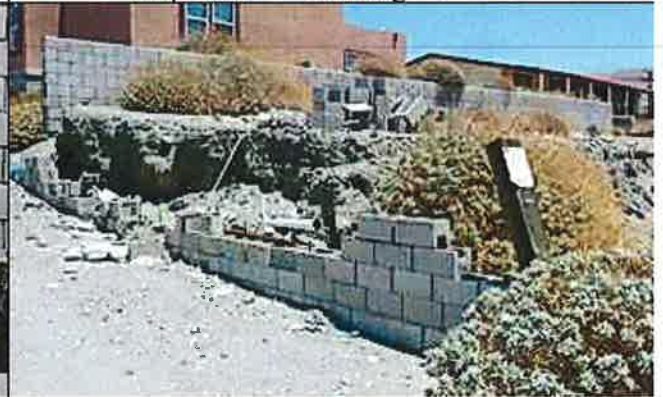
Unpermitted Grading 7/9/15 J. Cole
