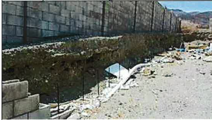
Cut Along the West Property Line and Block Wall 6/29/15 J. Cole
