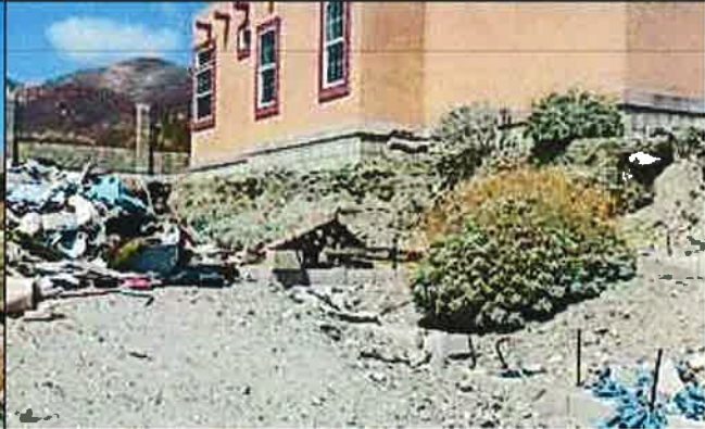
Substandard Structure 5/7/15 J. Cole
