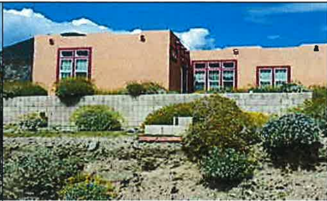
Substandard Structure 3/18/15 J. Cole
