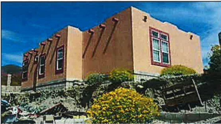
Substandard Structure 3/18/15 J. Cole
