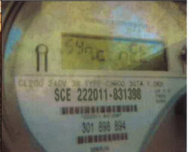
02/05/15 - Substandard Structure - NOD# 6,14,15 - Pike
