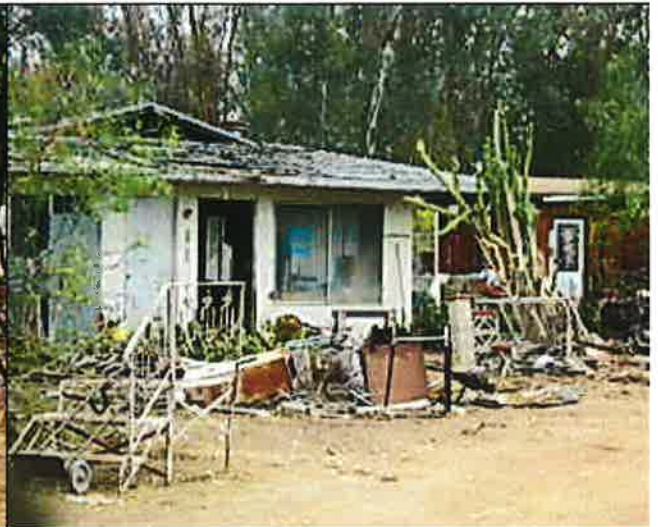
Structure remains substandard-JMorris 5/6/15
