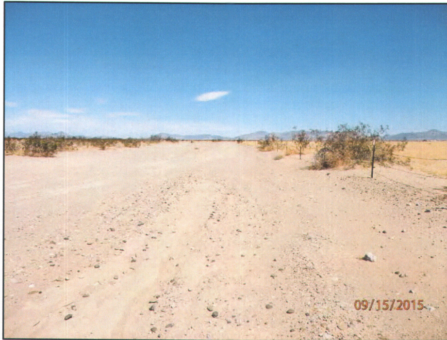
Photo 5 Access road and gen-tie line corridor along Butch Boulevard looking north toward solar facility (0.1 mile segment)
