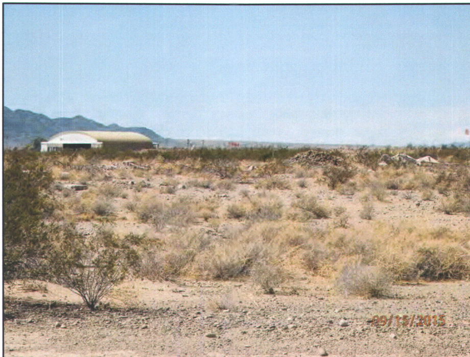
Photo 4 Interior patch with runway rubble
