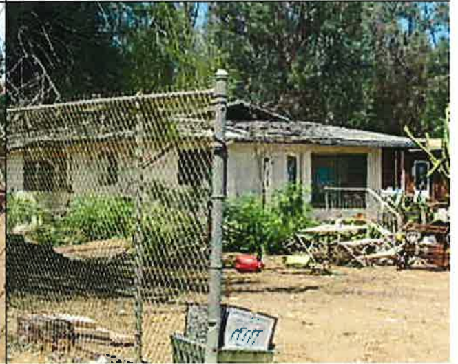
Structure remains substandard-JMorris 7/28/15
