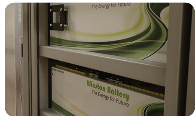
1MW Stationary Battery
