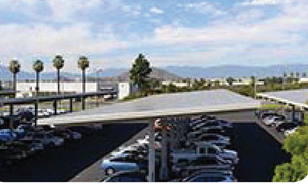
500 KW Solar Carport
