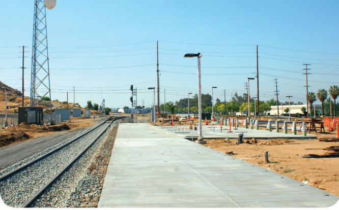
Hunter Park Metrolink Station currently under construction
