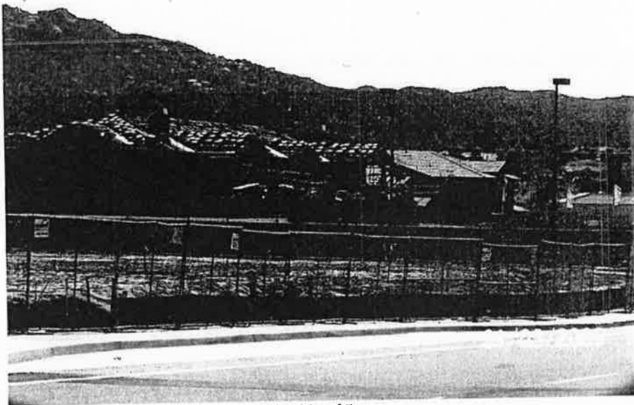
North Side of Property
