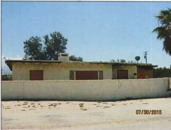
Property remains boarded up and clean. 1 of 3.
