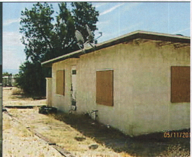
Structure now boarded up and cleaner. 1 of 8.
