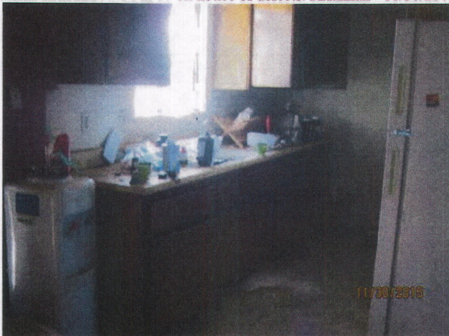
Inside structure'. # 14 & 17 on notice of defects. RHannah - 11/30/2015
