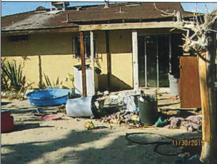
Accumulated rubbish/ trash, number 17 on notice of defects also.
